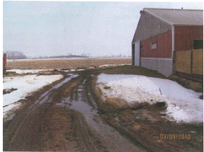
View toward heifer feedlot runoff discharge; flows off lot into low ditch area that is tiled.
