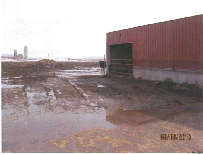
Photos above and below: Looking southeast/east, manure and roof water flushes through this area and discharges to road ditch.
