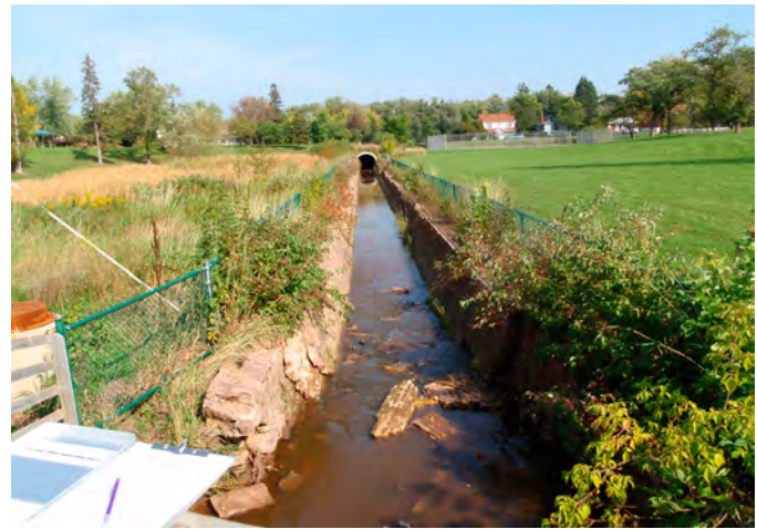
Faxon (Central Park) Creek – channelization
