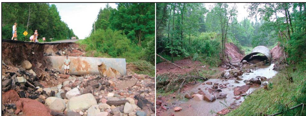
Figure 7: Examples of failed culverts in the soil transition zone of the Marengo River Watershed. Left photo by Diane Daulton, right photo by Bad River Watershed Association.
