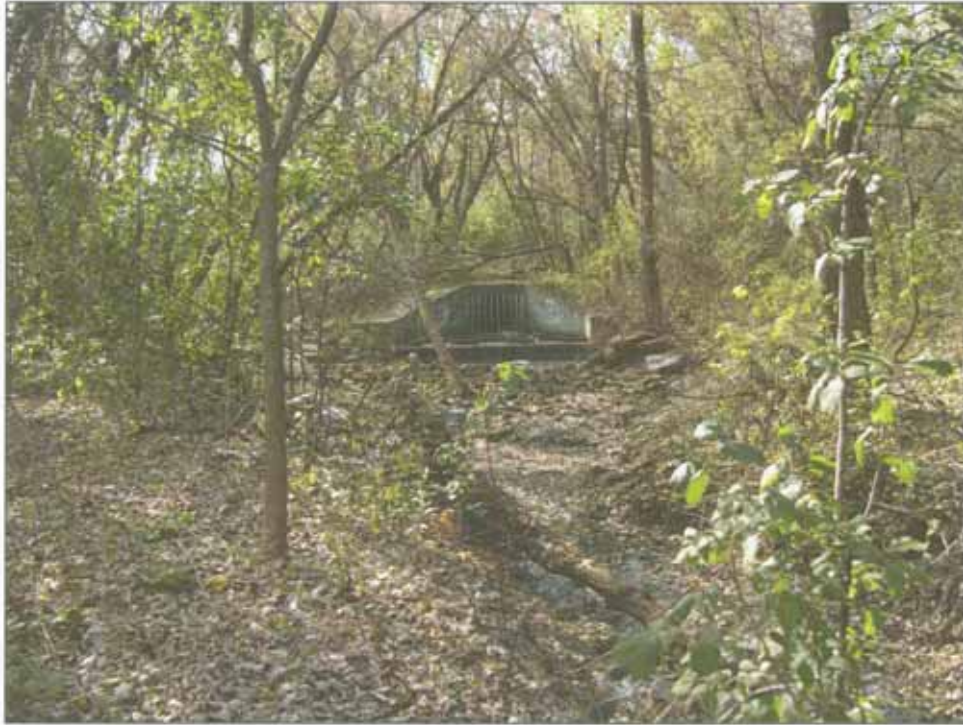
Stormwater culvert near S5, looking southwest
