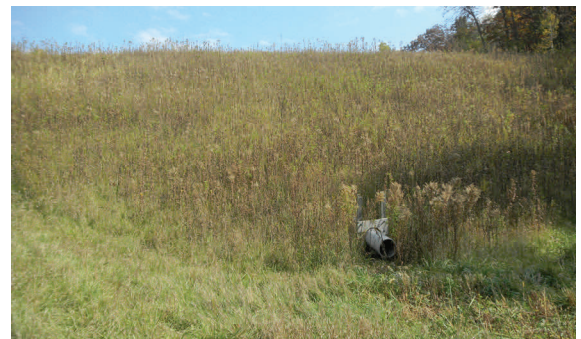
Erosion control structure with underdrain.
