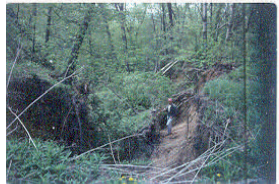
Gully erosion before stabilization.
