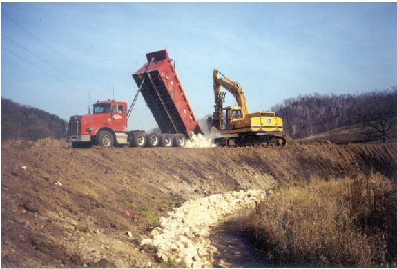
Installation of rip-rapping and stabilization of streambank.
