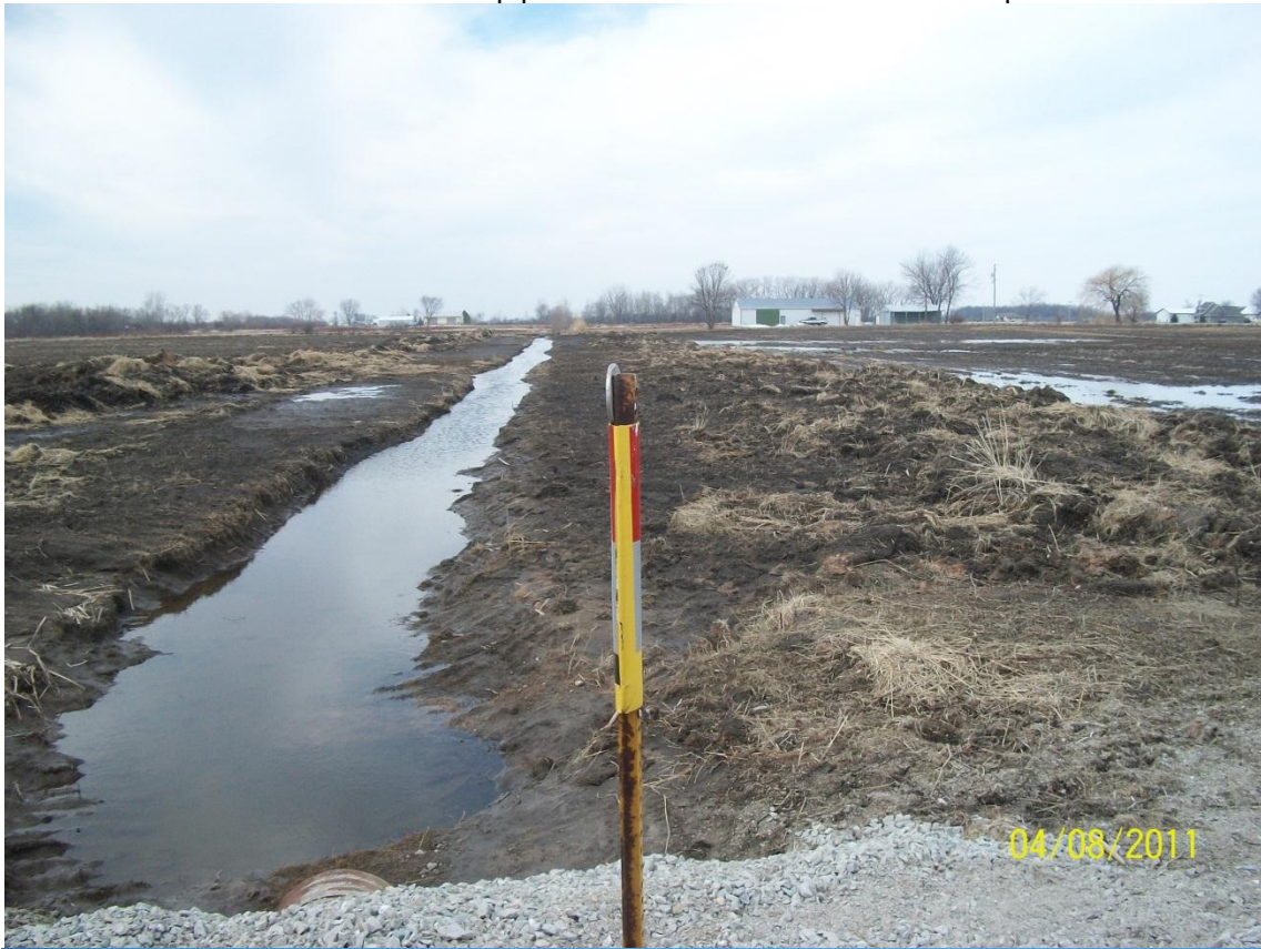
Before buffer installed top picture. After buffer installed bottom picture
