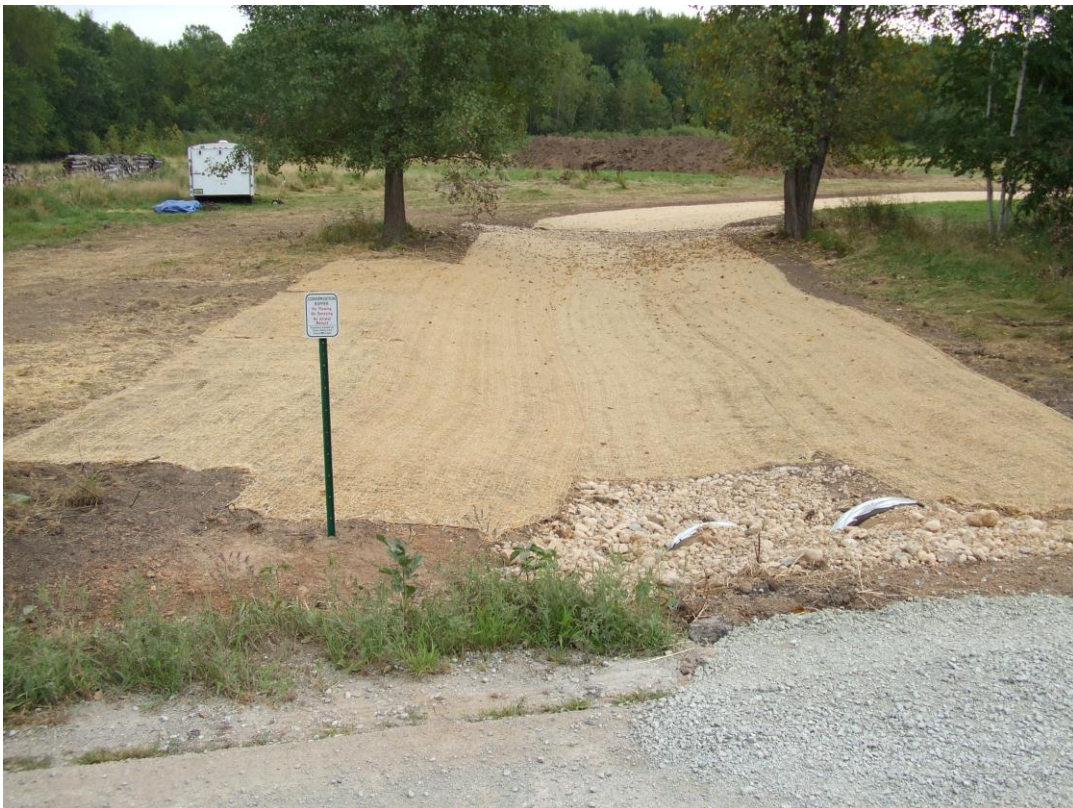
Erosion netting for buffer seeding
