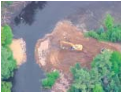
Thursday morning 6/7/01. Following drawdown, breaching, and channel relocation on the first two days, the contractor is preparing to widen the new channel to match the natural river width.
