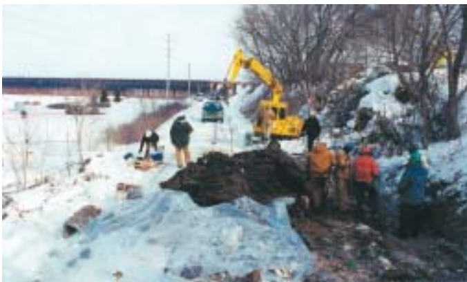
Cleanup of Ashland Coal Tar Site seep.
