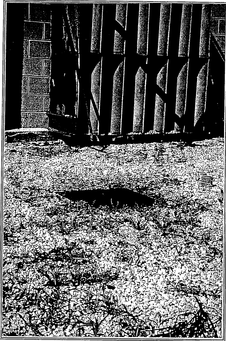
Description: Amcast Storm Sewer to be Sampled
