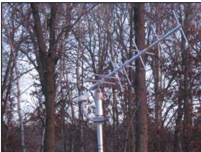
Close-up of antenna mast.
