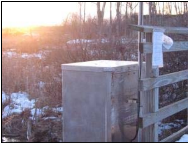
Rear of gage house (looking southwest).
