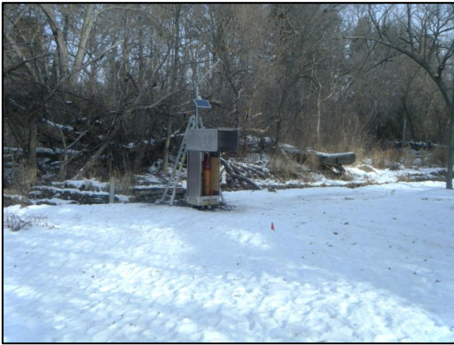
Gaging Station installed Jan 2013 along creek bank
