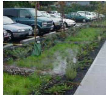
**Examples of stormwater managment.** These are images of rain gardens, vegetated swales, green roofs, and other BMPs that reduce the quantity and improve the quality of stormwater runoff in urban areas.
