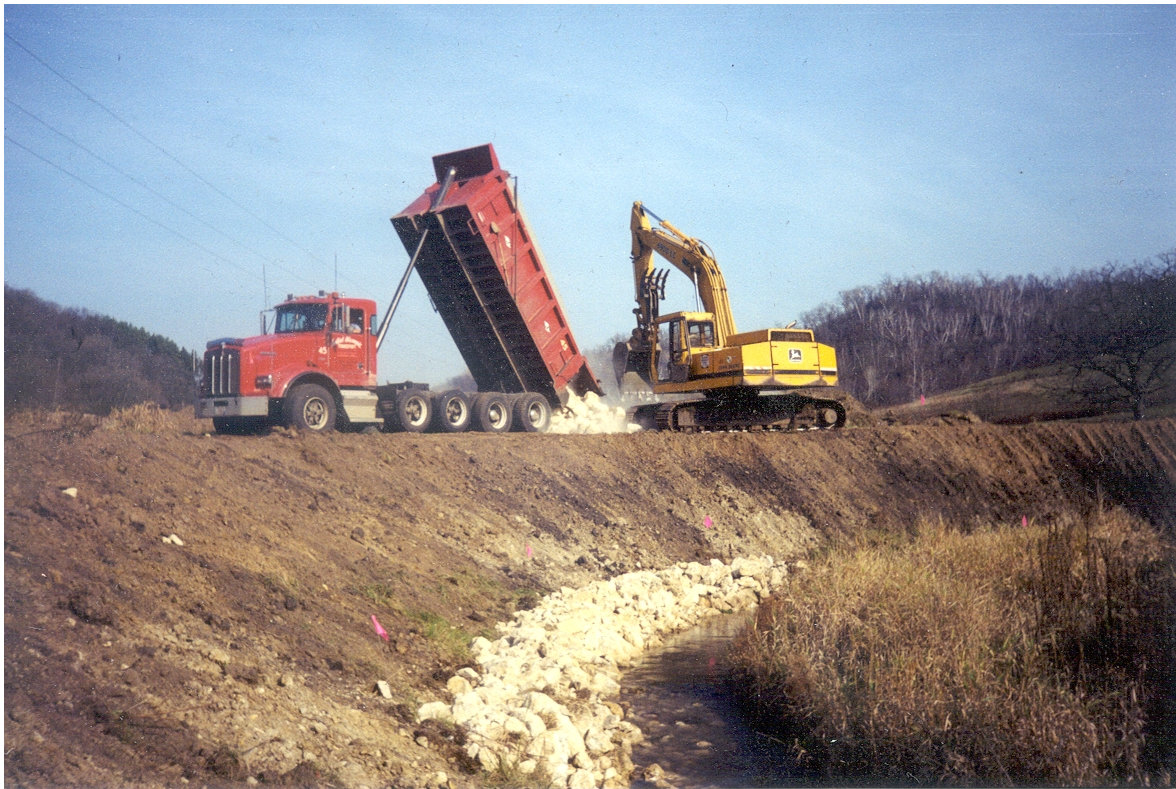
Installation of rip-rapping and stabilization of streambank
