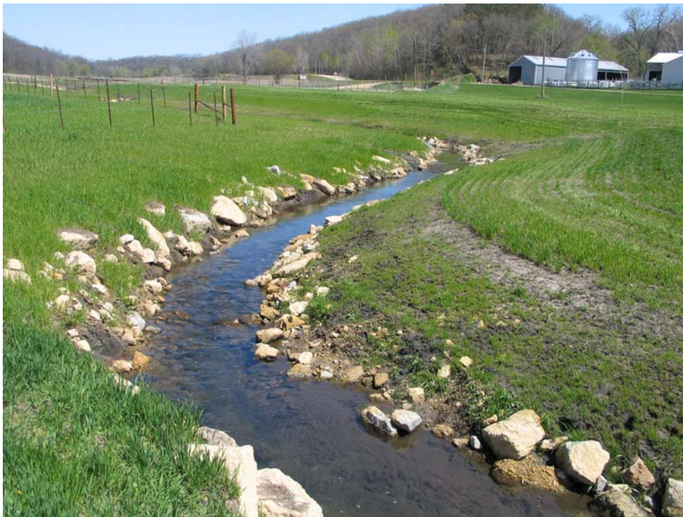
German Valley Creek after : Actually moved the stream back to its original bed and meander pattern and away from the barnyard. Filter bed put in. Fence to keep cattle out.
