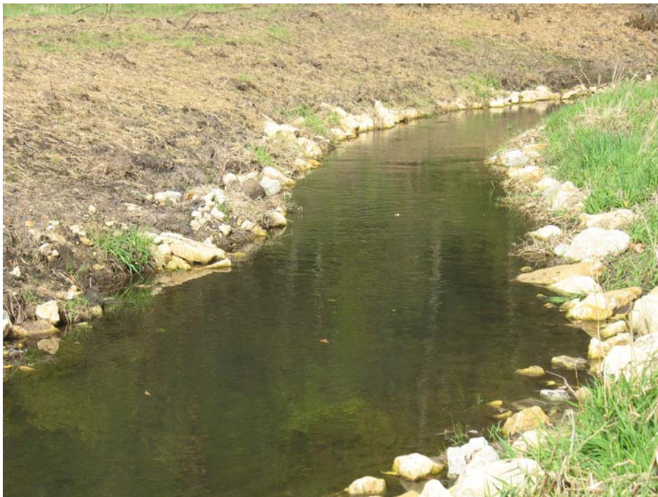
German Valley Creek after : Banks sloped, seeded, stabilized; stream able to spread out in high flow events, reducing erosive energy.
