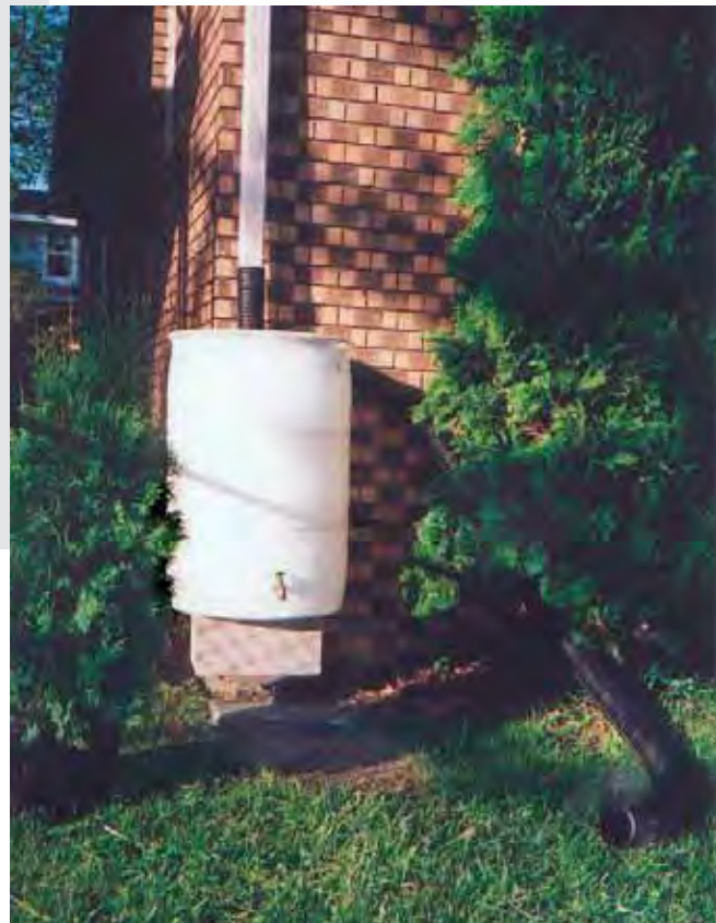
Figure 5-1. Rain barrel. (Courtesy of the River Alliance of Wisconsin.)
