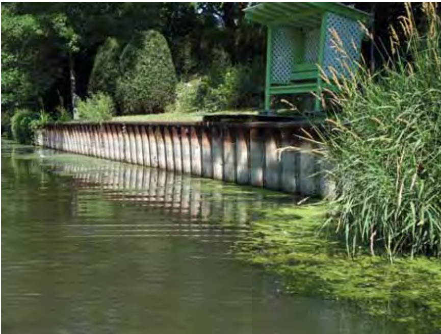
Figure 2-7. Corrugated steel piling sheets serving as armor on the lower West Branch.
