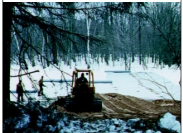
Figure 1. Spreading Geotextile over Frozen Lake
