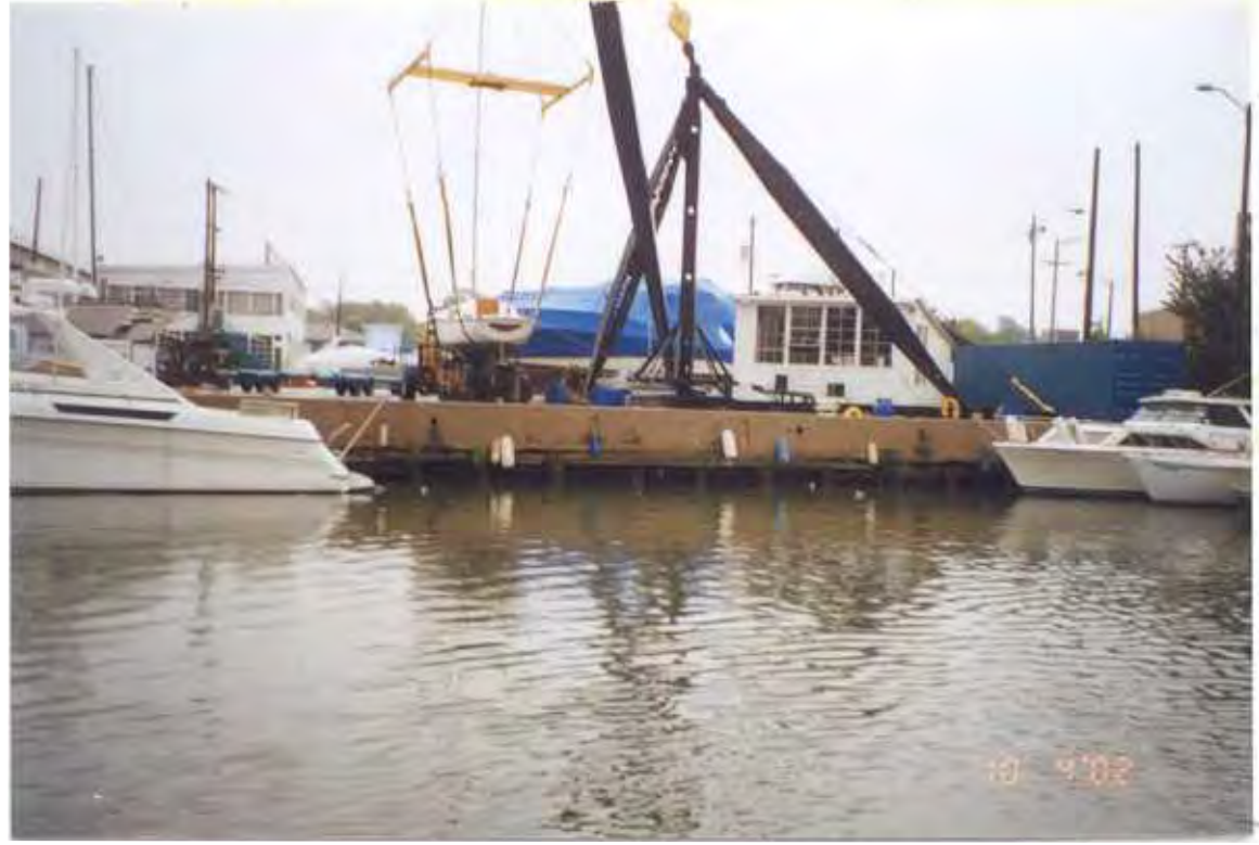
PHOTO 28 – October 4, 2002 – Kinnickinnic River Taken by Tor Hansen, Barr Engineering Concrete dock and timber wall at Parcel 426A. Looking north.
