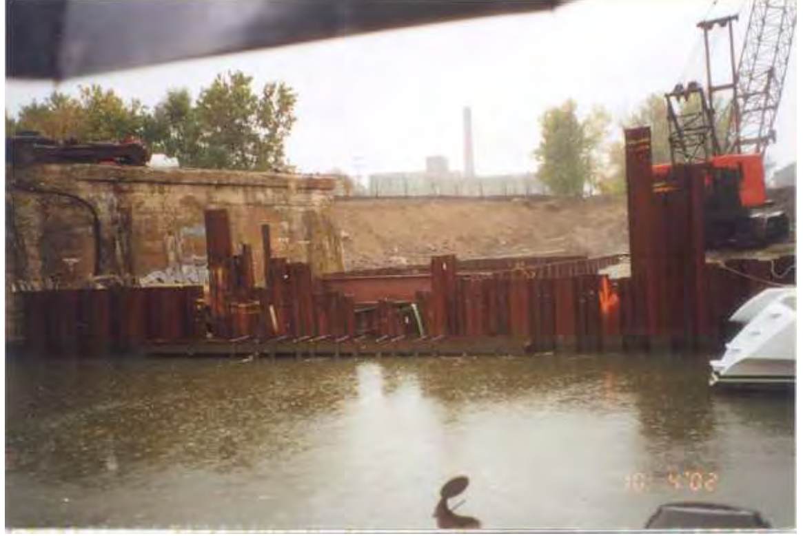
PHOTO 68 – October 4, 2002 – Kinnickinnic River Taken by Tor Hansen, Barr Engineering New steel sheet pile construction adjacent to old bridge abutment at Parcel 440. Looking south.
