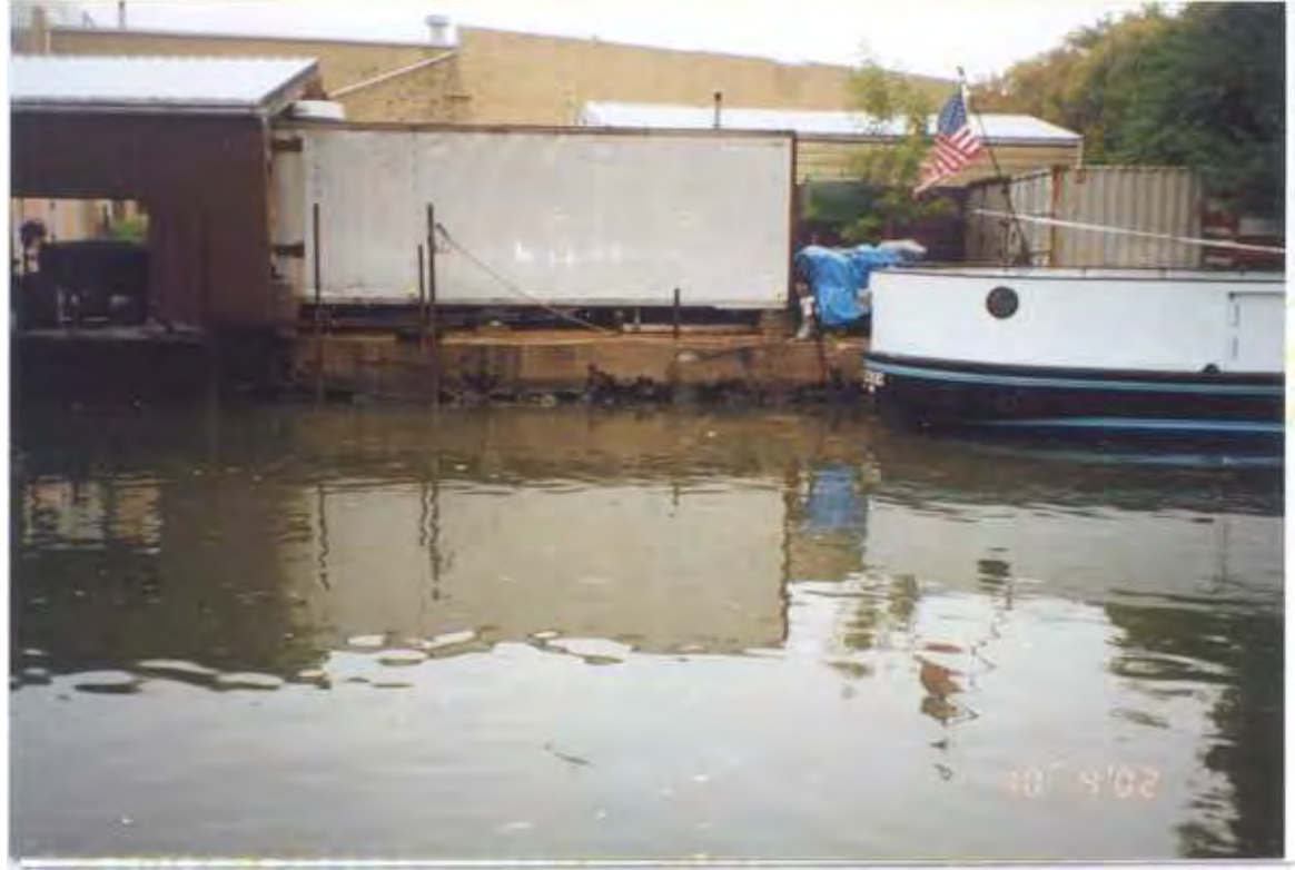
PHOTO 36 – October 4, 2002 – Kinnickinnic River Taken by Tor Hansen, Barr Engineering Concrete and timber wall along Parcel 425. Looking north.
