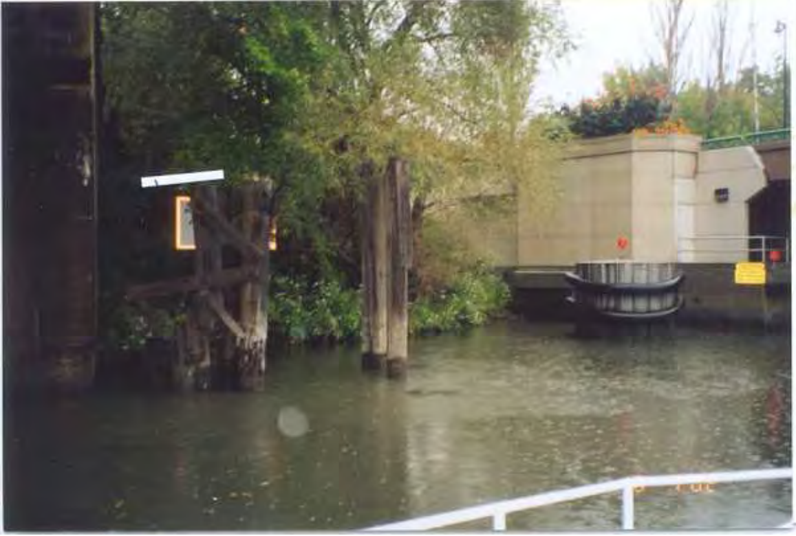
PHOTO 42 – October 4, 2002 – Kinnickinnic River Taken by Tor Hansen, Barr Engineering Vegetation at shoreline upstream from Kinnickinnic Avenue left bridge abutment. Looking north.
