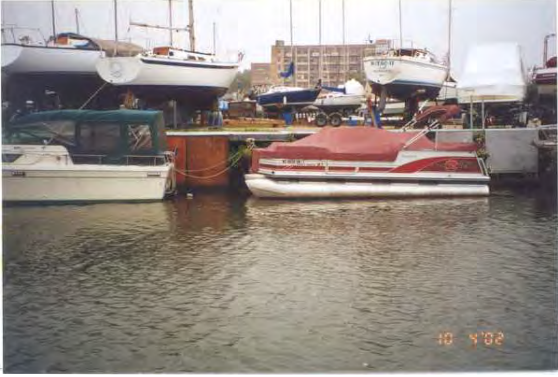
PHOTO 21 – October 4, 2002 – Kinnickinnic River Taken by Tor Hansen, Barr Engineering Timber dock and wall along Parcel 426B. Looking north.
