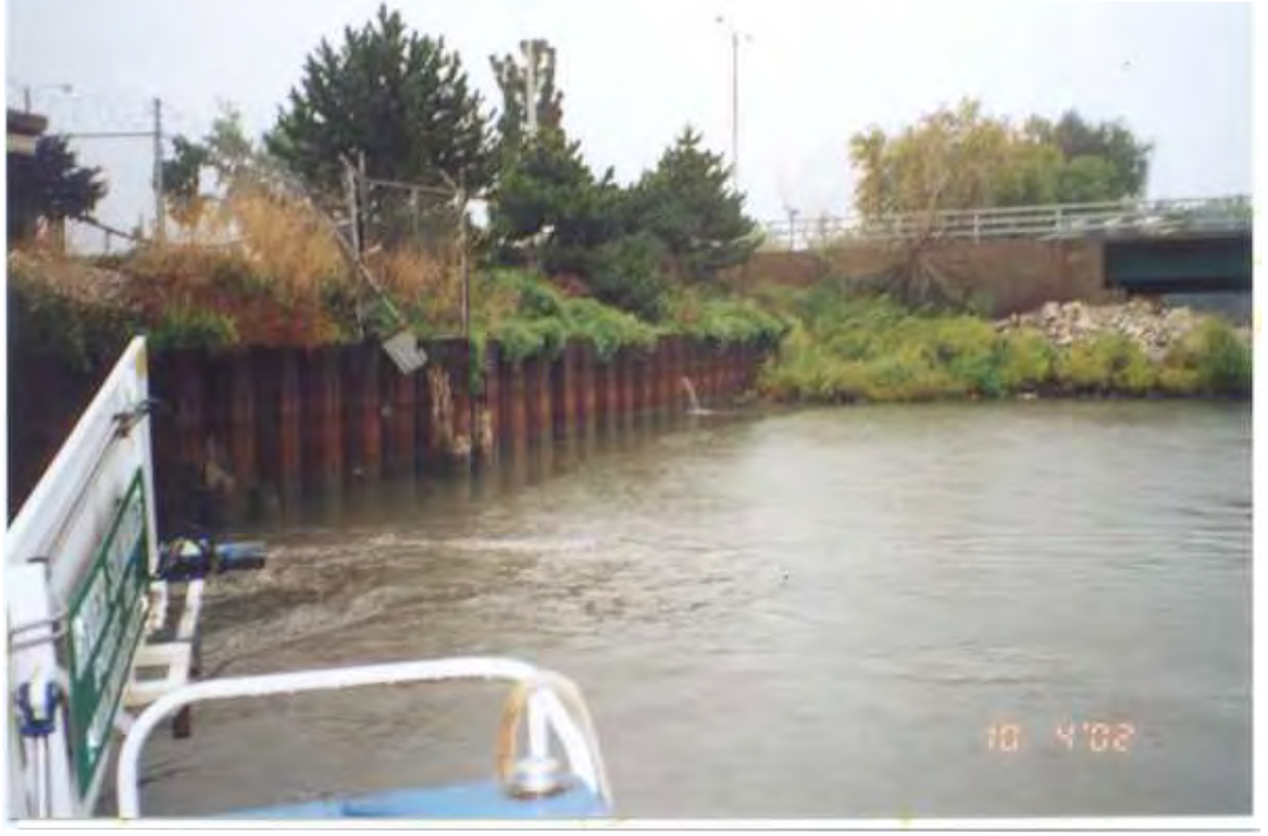
PHOTO 47 – October 4, 2002 – Kinnickinnic River Taken by Tor Hansen, Barr Engineering Steel sheet pile wall along Parcel 432 and upstream end of Steel sheet pile wall along Parcel 433. Looking southeast.
