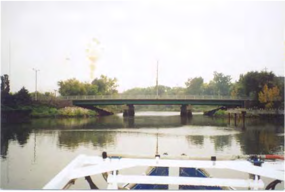
PHOTO 1 – October 4, 2002 – Kinnickinnic River Taken By Tor Hansen, Barr Engineering Becher Street Bridge looking upstream (South)
