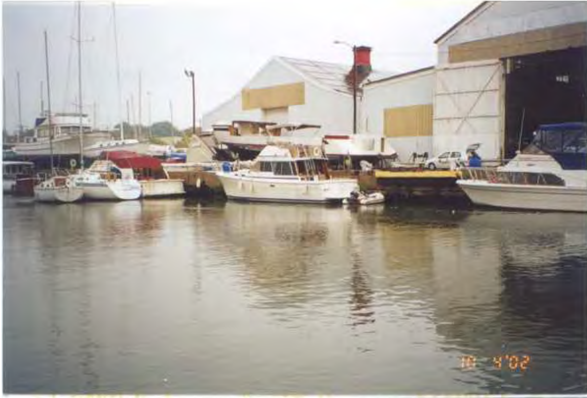
PHOTO 26 – October 4, 2002 – Kinnickinnic River Taken by Tor Hansen, Barr Engineering Concrete dock and timber wall at Parcel 426A. Looking north.
