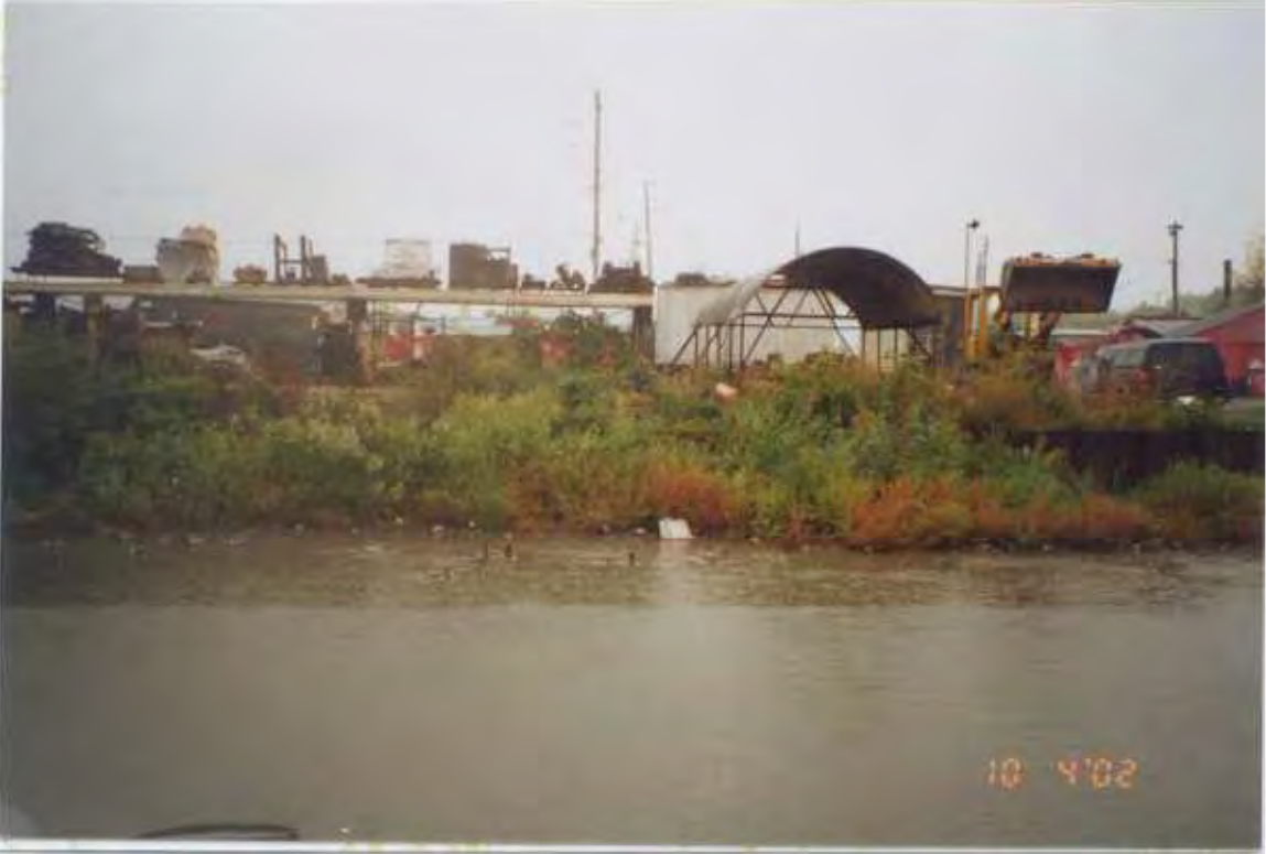
PHOTO 58 – October 4, 2002 – Kinnickinnic River Taken by Tor Hansen, Barr Engineering Downstream end of steel sheet pile wall at Parcel 433 and start of vegetation along Parcel 436. Looking south.
