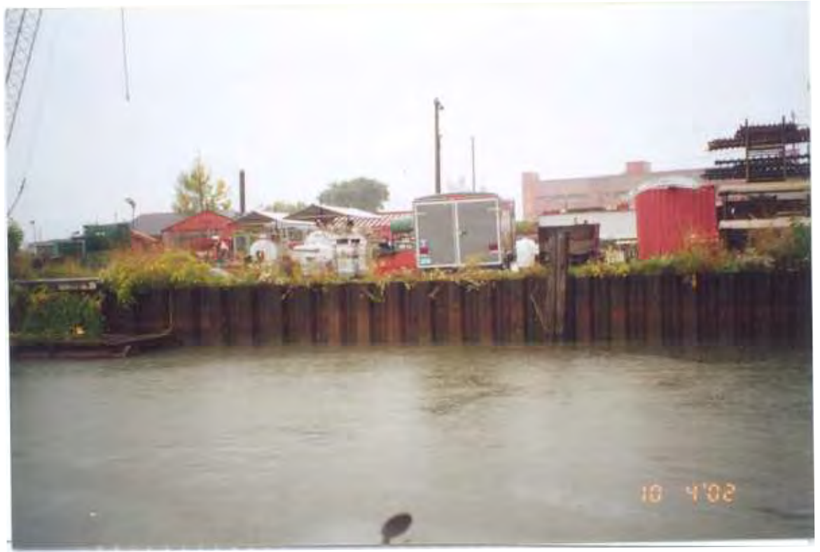
PHOTO 52 – October 4, 2002 – Kinnickinnic River Taken by Tor Hansen, Barr Engineering Steel sheet pile wall along Parcel 433. Looking east.
