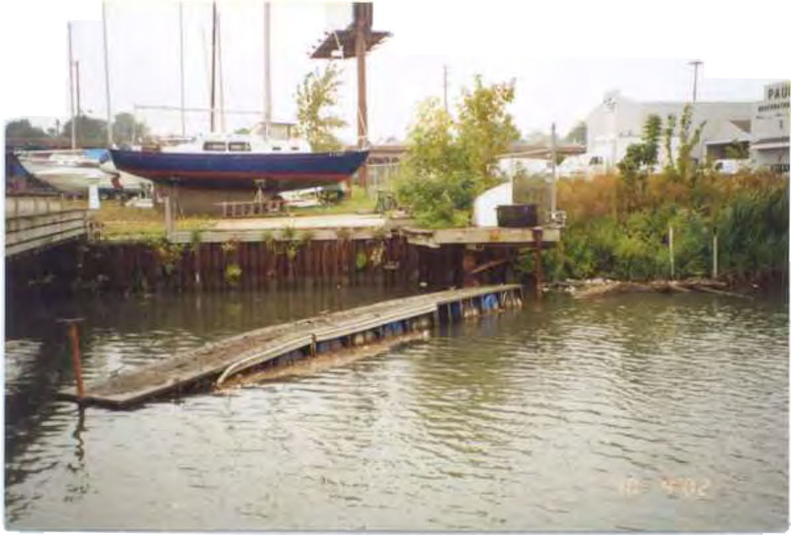
PHOTO 10 – October 4, 2002 – Kinnickinnic River Taken by Tor Hansen, Barr Engineering Downstream end of steel sheet pile wall along Parcel 429 and upstream end of Parcel 428 showing vegetative cover at shoreline. Looking west.
