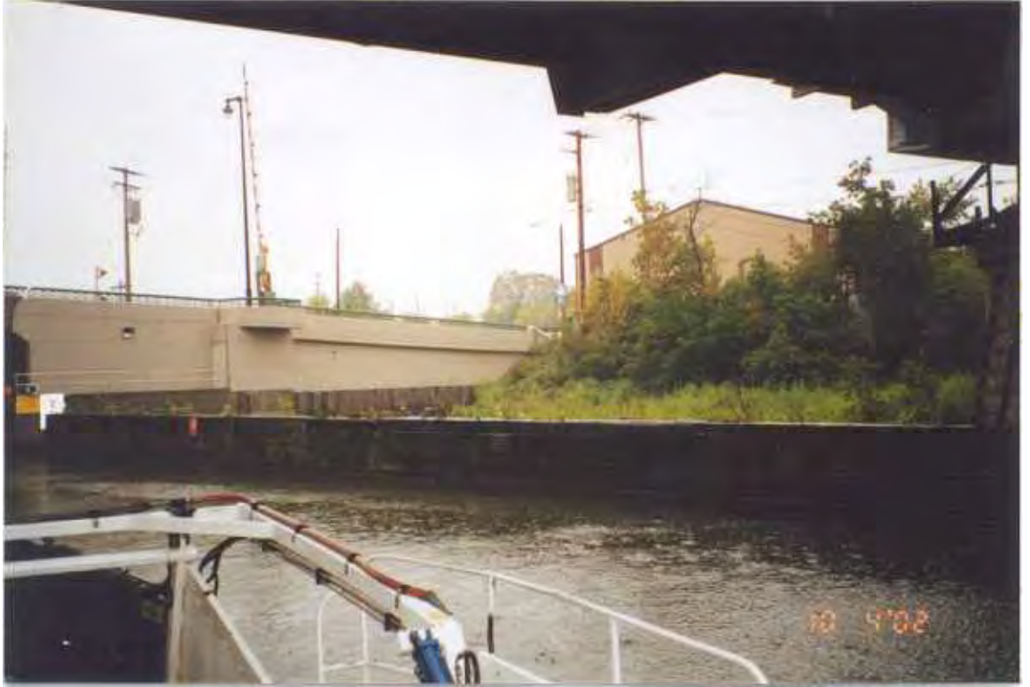
PHOTO 72 – October 4, 2002 – Kinnickinnic River Taken by Tor Hansen, Barr Engineering Timber pile fence protecting bridge pier adjacent to Parcel 443. Looking south.
