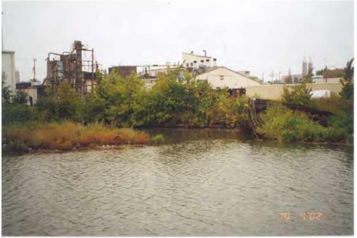
PHOTO 15 – October 4, 2002 – Kinnickinnic River Taken by Tor Hansen, Barr Engineering Vegetation and old timber wall in corner of Parcel 427. Looking north.
