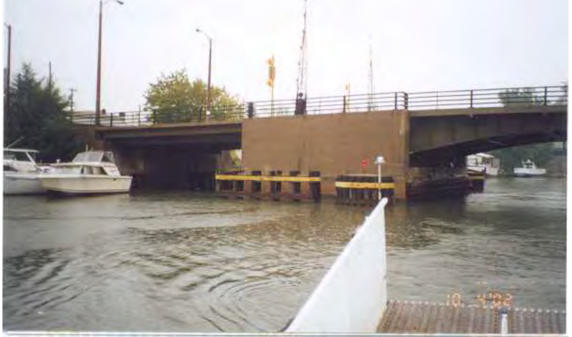
PHOTO 44 – October 4, 2002 – Kinnickinnic River Taken by Tor Hansen, Barr Engineering Upstream face of left abutment and pier of 1 st Street Bridge. Looking downstream or east.
