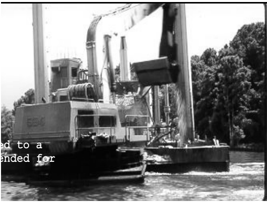
Computer Controlled Dredging Source: U.S. EPA Region 6
