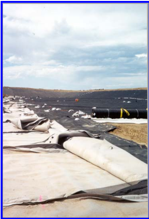
Liner Installation for Disposal Site Source: ThermoRetec
