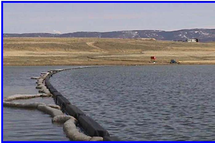
Silt Curtain Source: ThermoRetec
