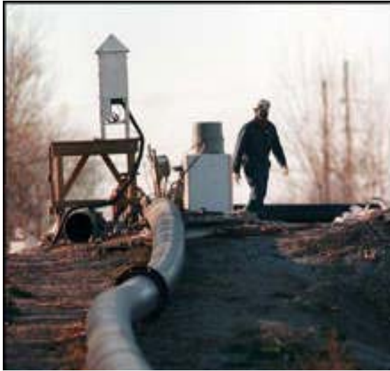
Air Monitoring Equipment Source: B. Paulson, WDNR
