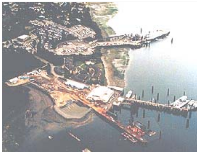
Construction of Nearshore Fill CDF Source: U.S. EPA
