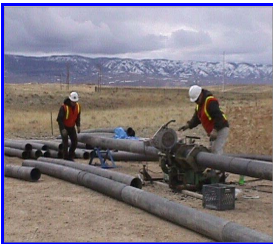
Assembling Slurry Pipeline Source: ThermoRetec
