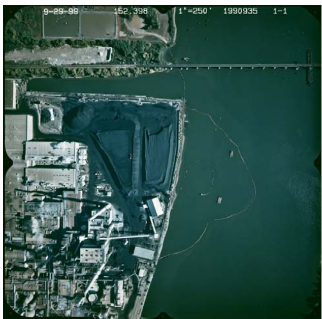
Aerial View of Silt Curtain and Dredge Source: B. Paulson, WDNR
