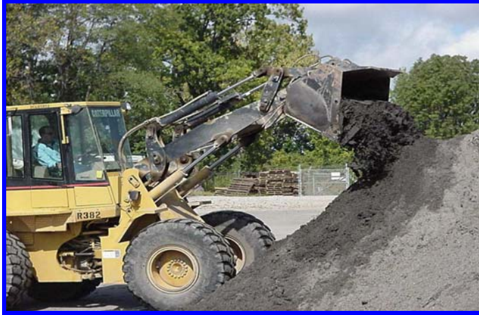
Stockpiling Dewatered Sediment Source: Bill Fitzpatrick, WDNR
