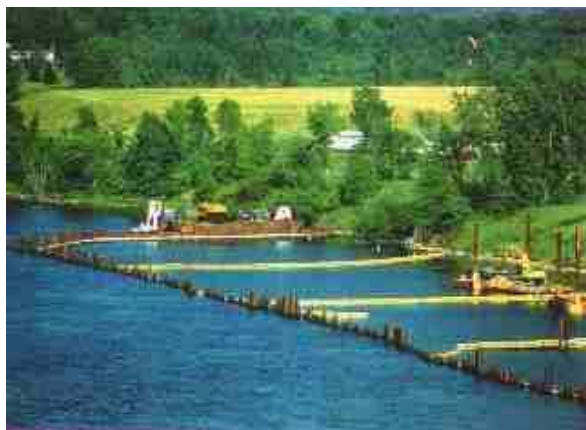
Dredging in St. Lawrence Source: K. Martin
