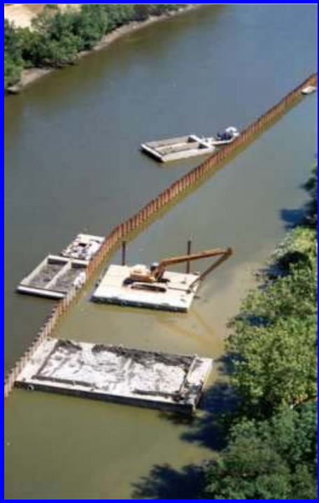
Christina River Dredging Source: Severson
