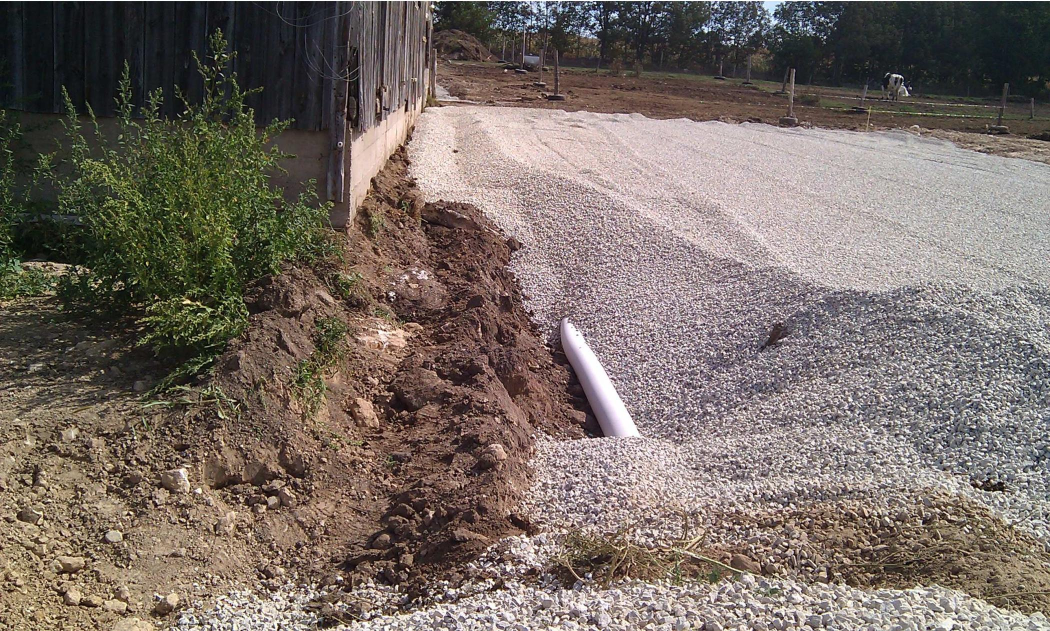
Ground Gutter for Roof Water
