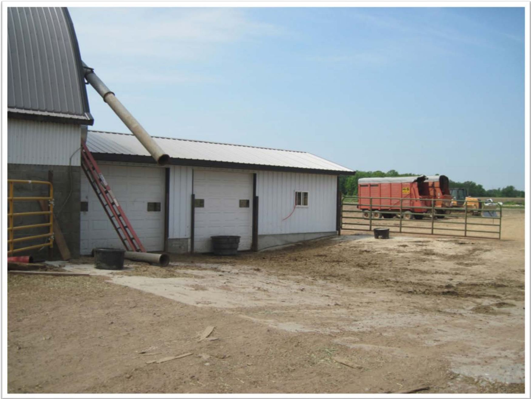
May 24, 2012 – Standing on the north side of the barn looking southwest at the machinery crossing installed to carry feedlot runoff water from the heifer/dry cow lot to the manure storage transfer so that it can be pumped to the manure storage facility.
