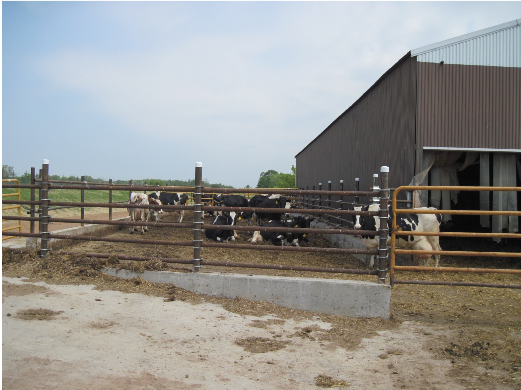
May 24, 2012 – Standing on the machinery crossing on the southwest side of the of the dry cow/heifer lot looking north. You can see between the east wall of the lot and the west side of the building there is a tiled rock envelop designed to catch any roof runoff and transport it underground to the waterway north of the machine shed.
