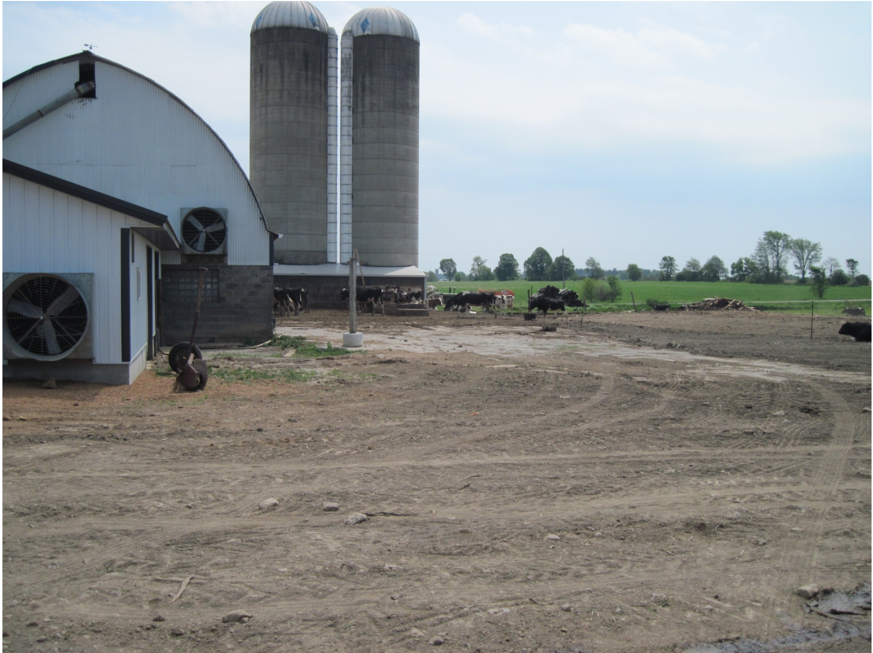
May 24, 2012 – Standing on the west side of the barn looking east, southeast over the area where the failing manure storage facility has been closed.
