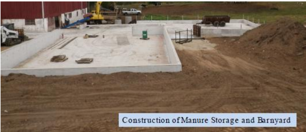
Construction of Manure Storage and Barnyard
