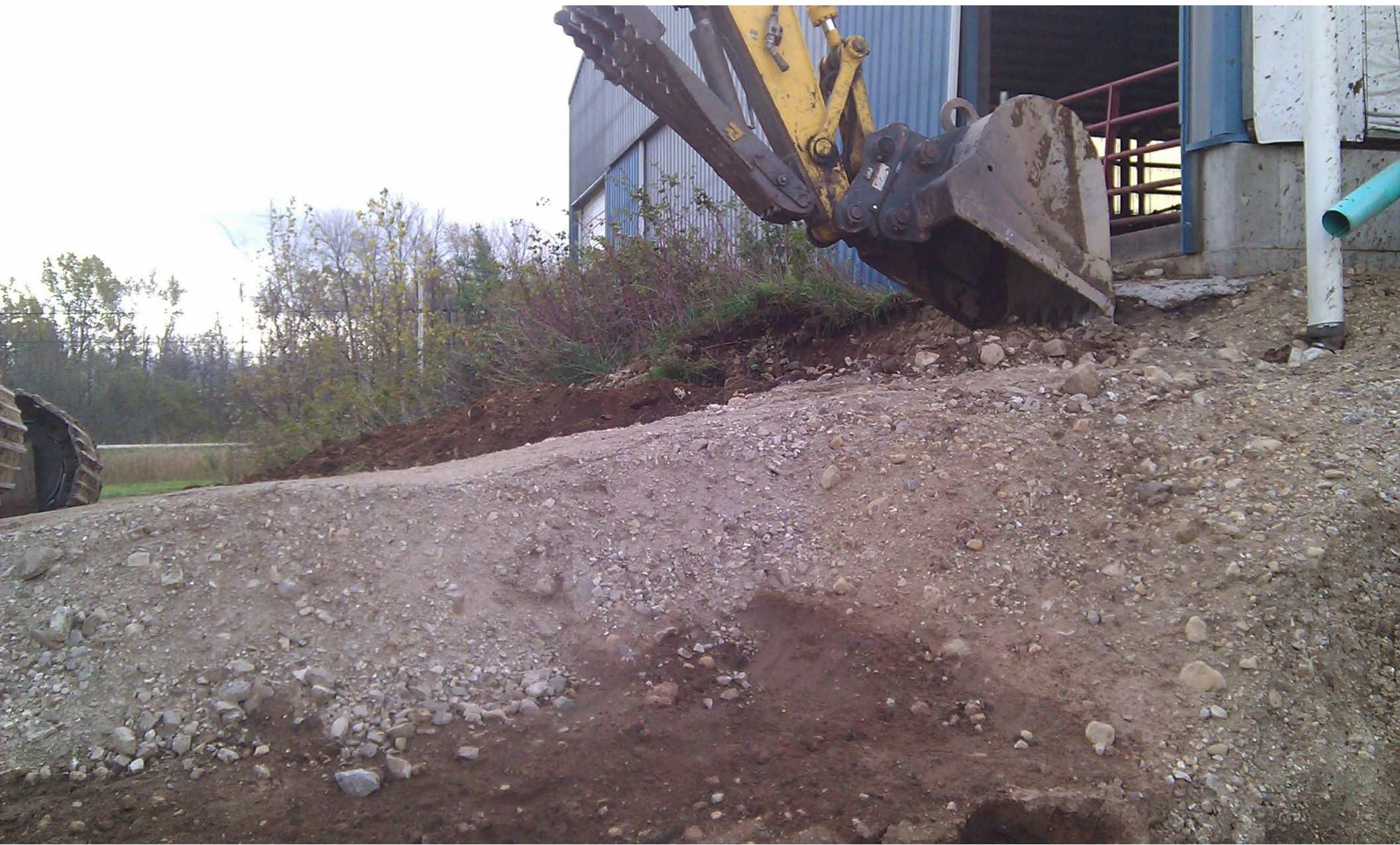
Excavation of Existing Reception Tank
