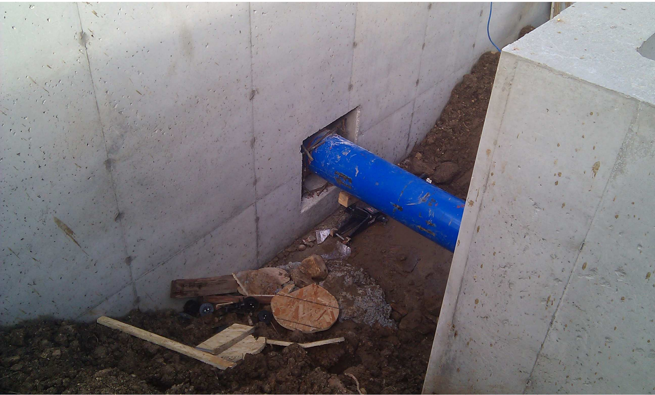
Waste Transfer Between Reception Tank and Manure Storage
