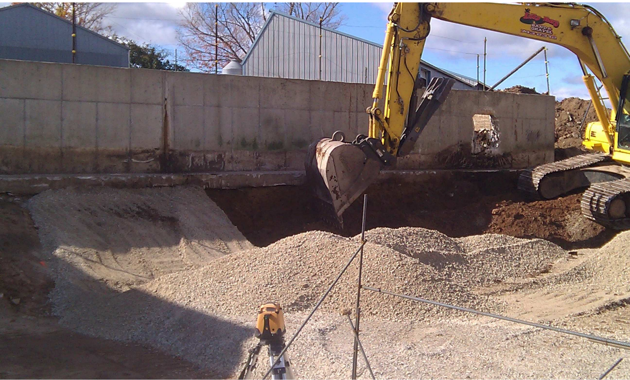
Excavation Adjacent to Existing Manure Storage
