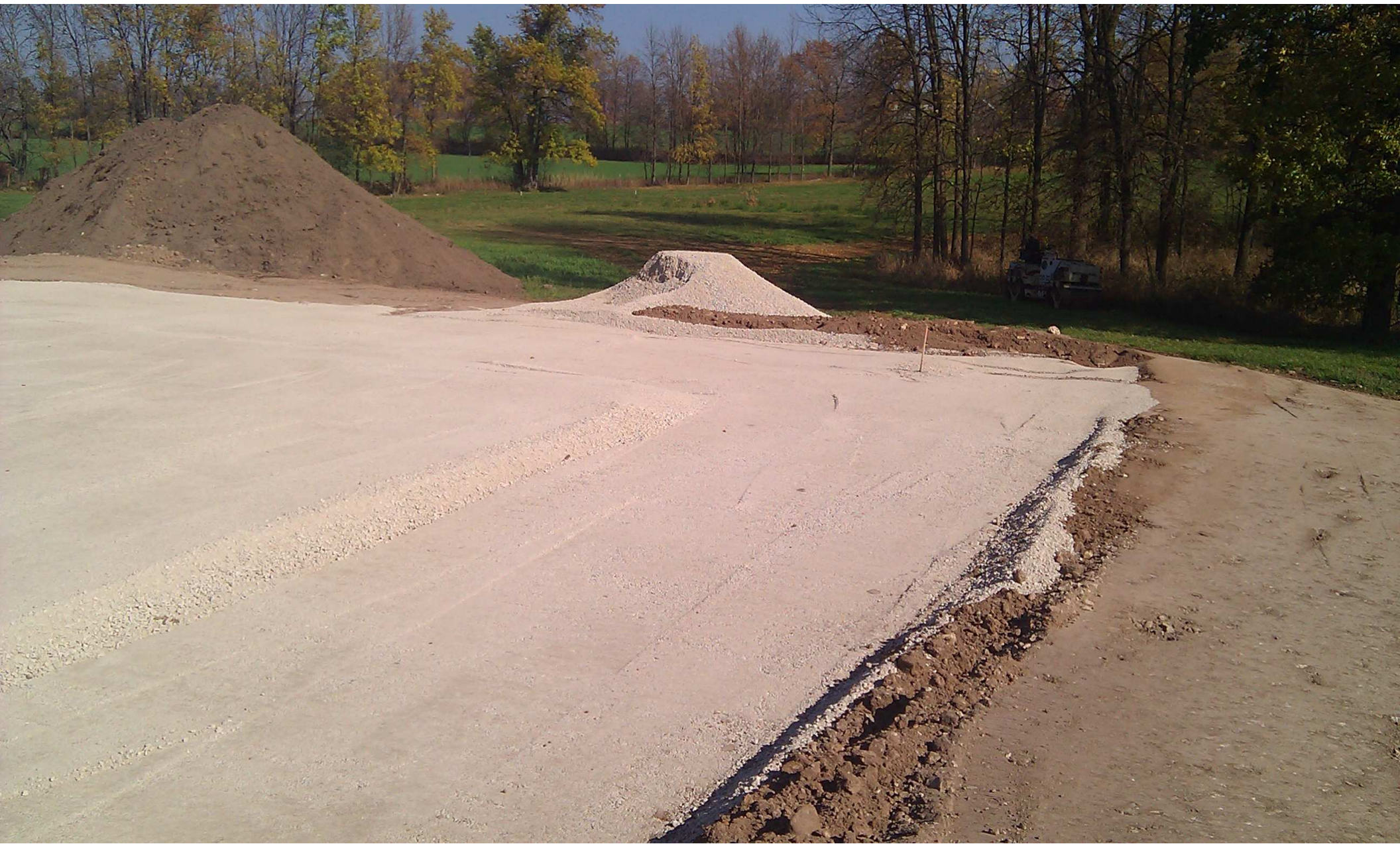
Preparation of Subgrade for Manure Storage
