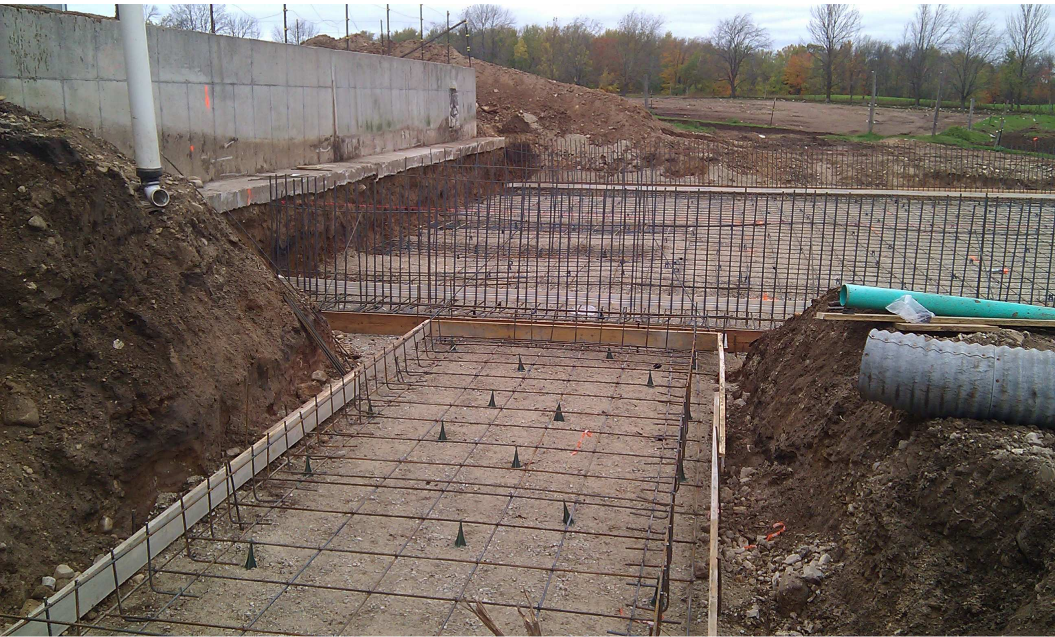
Construction of Reception Tank and Manure Storage
