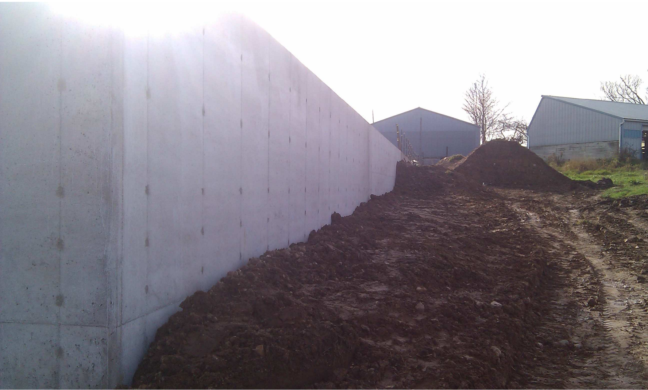
Backfilling of Manure Storage
