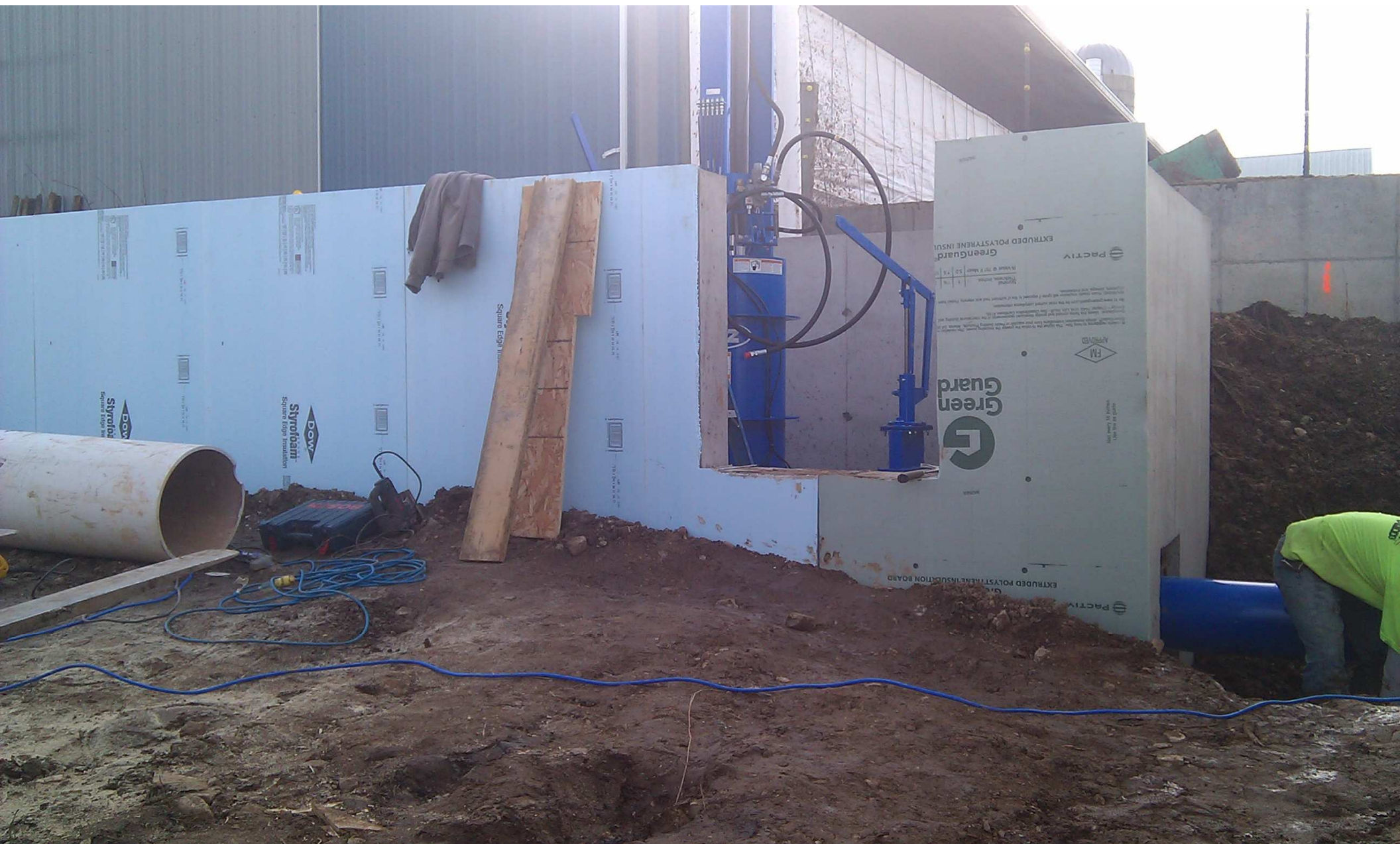
Manure Pump for Waste Transfer to Manure Storage
