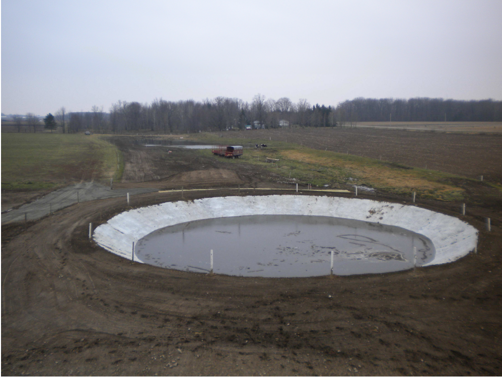
Complete Waste Storage Facility With Fence – Concrete Lined
