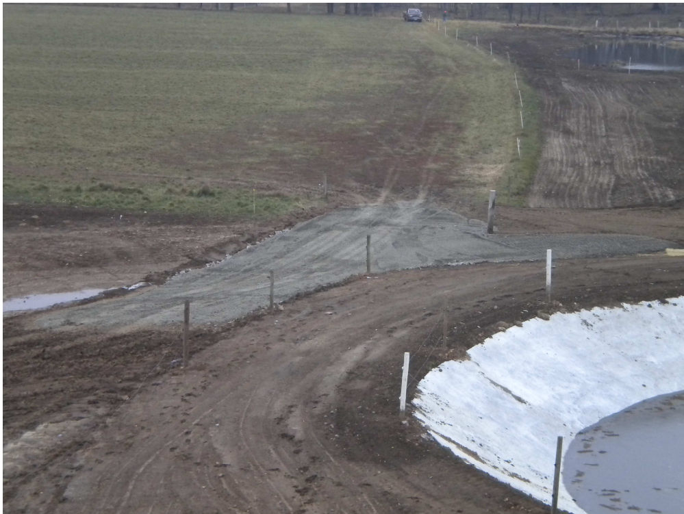
Picture of Diversion Ditch Crossing Behind The Pit
