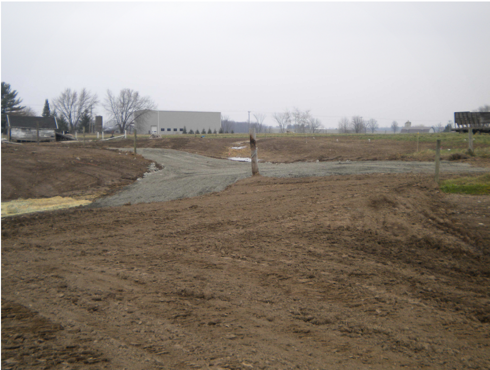
Diversion Crossing Looking At Diversion Ditch Upstream
