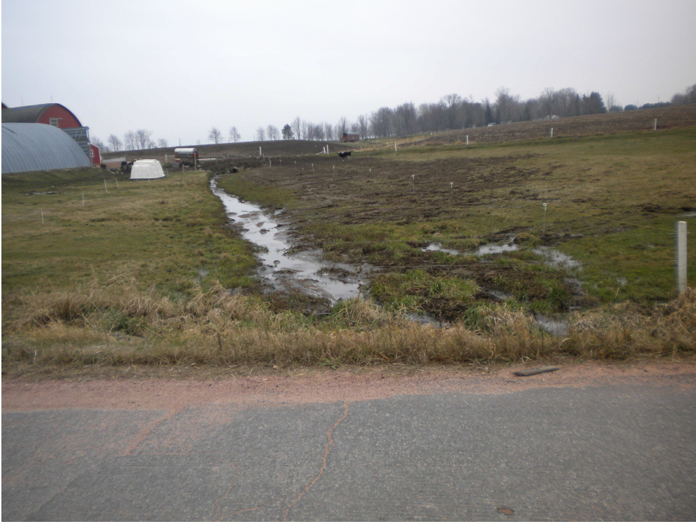
Ditch Viewing Upstream From Road – Fenced Out & Cattle Removed
