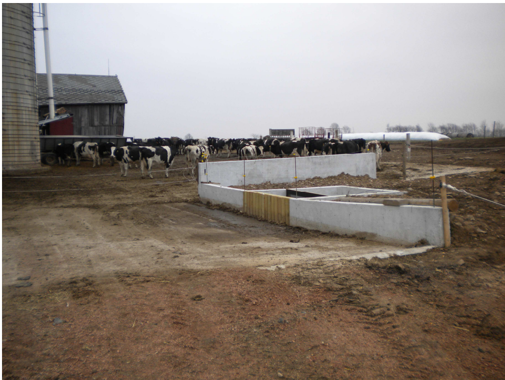
Another View Of Barnyard Settling Basin Area
