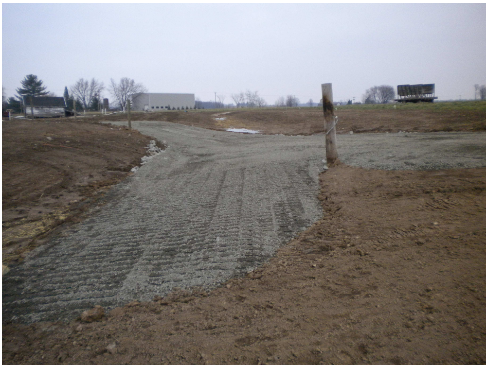
Picture of Diversion Ditch Crossing For Machinery
