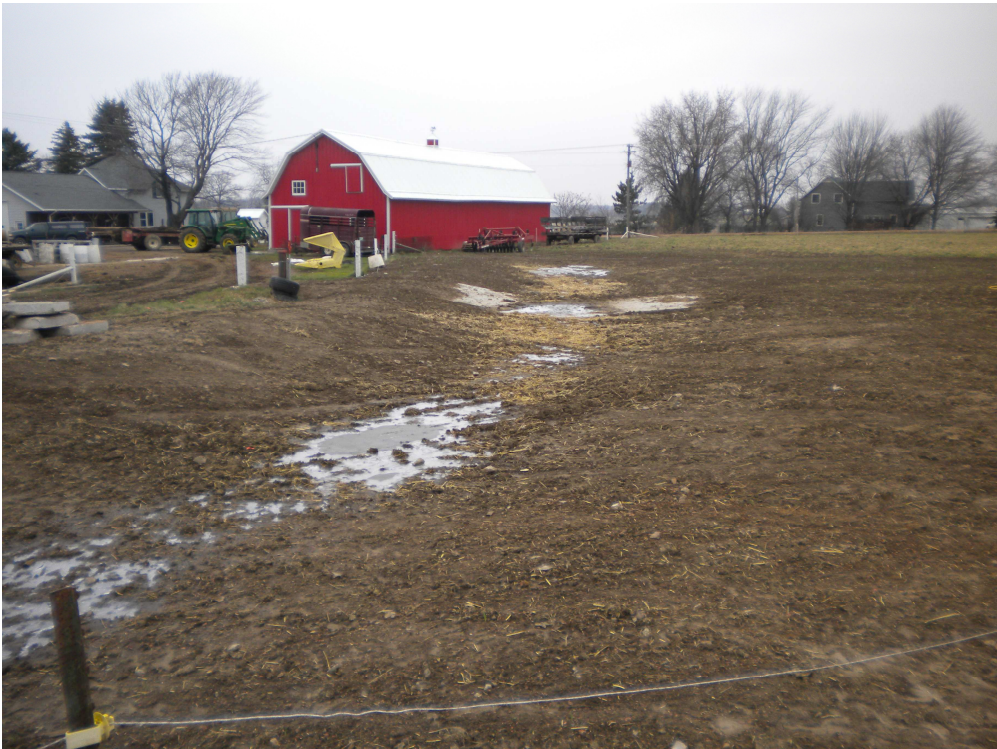
Another Diversion Crossing Looking At Diversion Ditch Upstream
