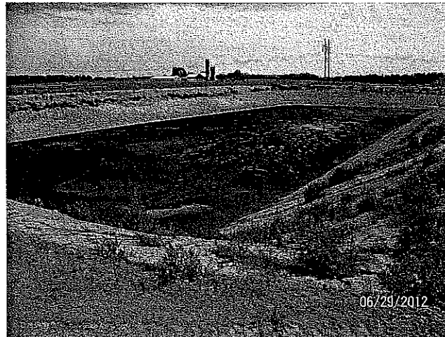
After - Expanded storage for adequate leachate storage
