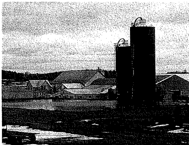
Before – Site with inadequate storage for leachate
