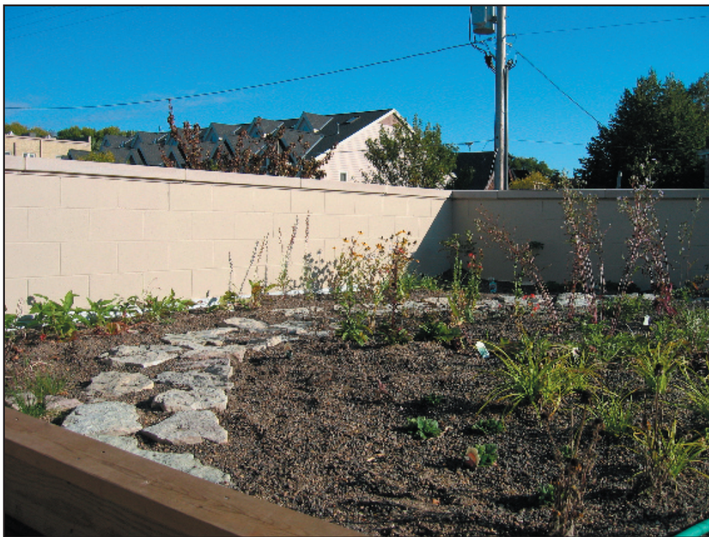
Figure 13: Green roof planting at Urban Ecology Center, Milwaukee, WI. Source Cheryl Bauer-Armstrong.
