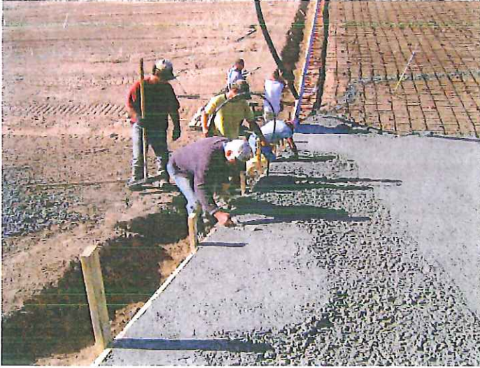
WATERSTOP AND CONCRETE VIBRATING OF WATERSTOP
