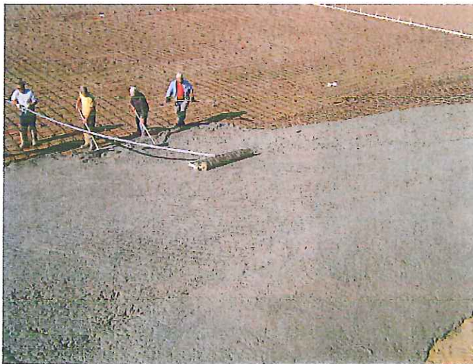
ROLLER BUGGY USED TO CONSOLIDATE CONCRETE
