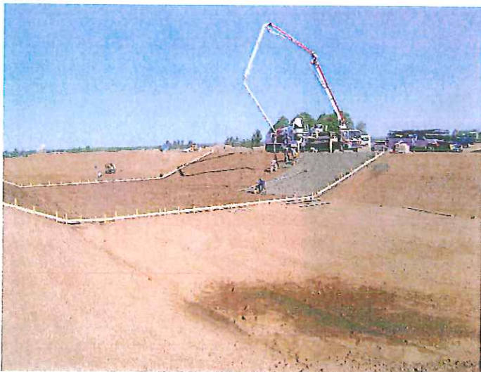
CONCRETE PUMPED IN PIT
