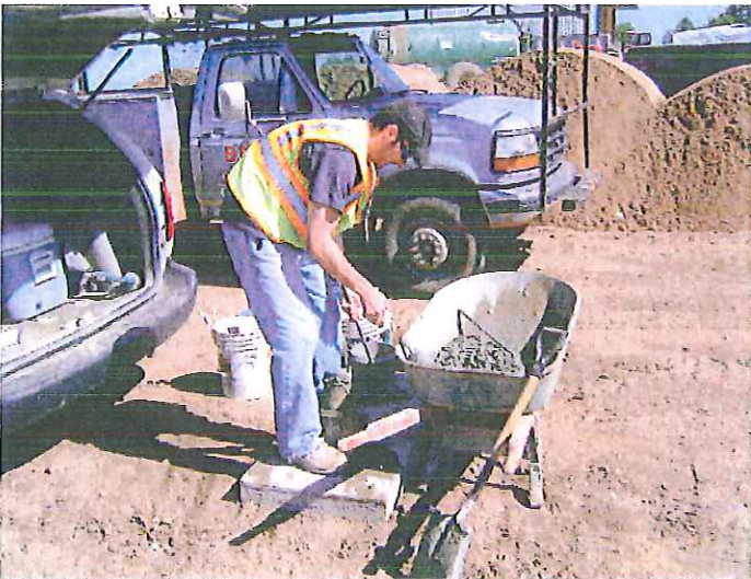
SLUMP TEST PERFORMED BY CONCRETE SUPPLIER
