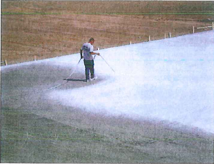
CURING COMPOUND APPLIED TO CONCRETE
