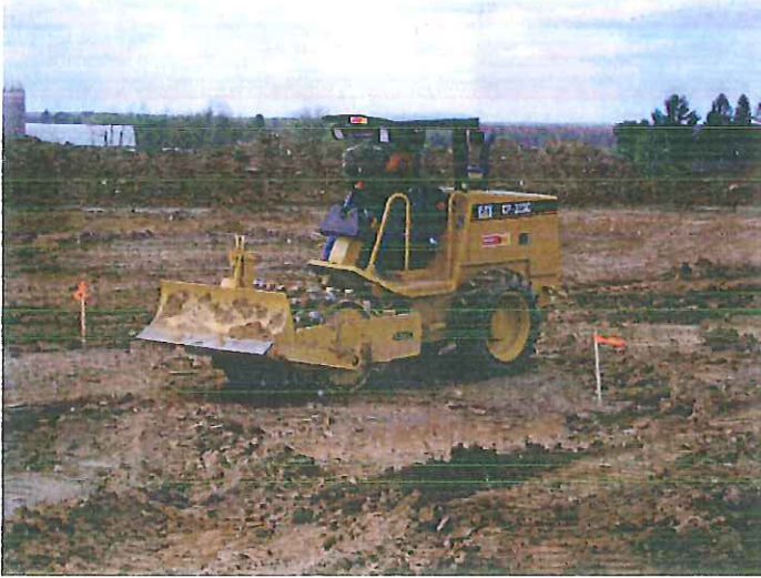
SHEEPS FOOT ROLLER FOR COMPACTING
