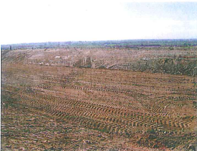
COMPACTING MANURE STORAGE FLOOR
