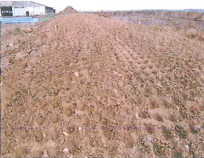
NORTH BERM COMPACTION
