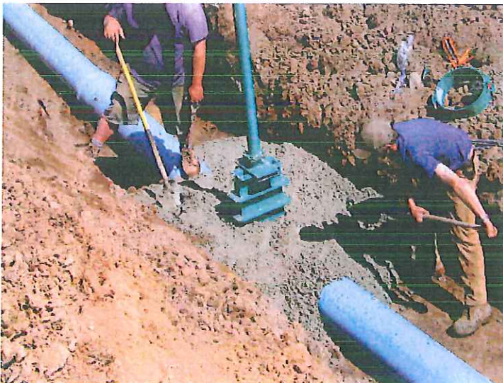
THRUST BLOCK FOR GATE VALVE
