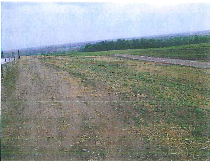
TOP SOIL REAPPLIED, SEEDED, AND MULCHED
