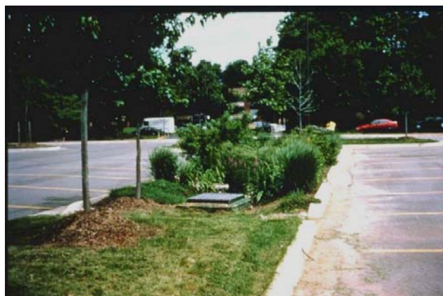
BIOFILTER IN PARKING LOT
