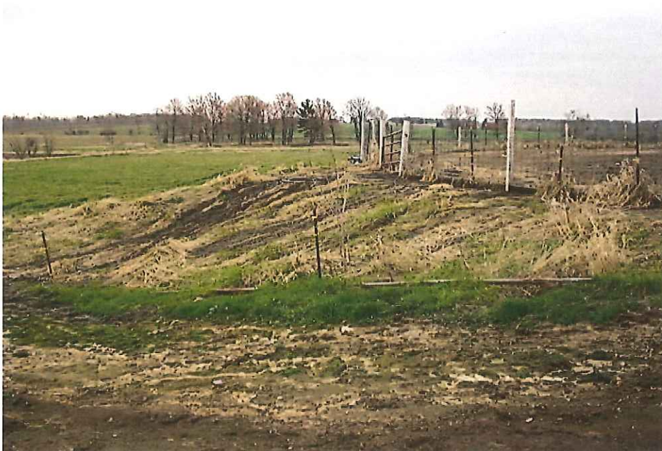
Over flowing waste storage facility
