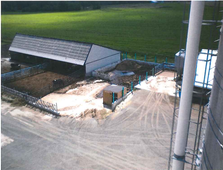
Feet lot #1 – Heavy use protection stacking area to scrape upper young stock housing and barnyard scrapings. The liquids and some solids are collected in a reception tank under the barnyard and pumped to long term storage. Zero discharge.
