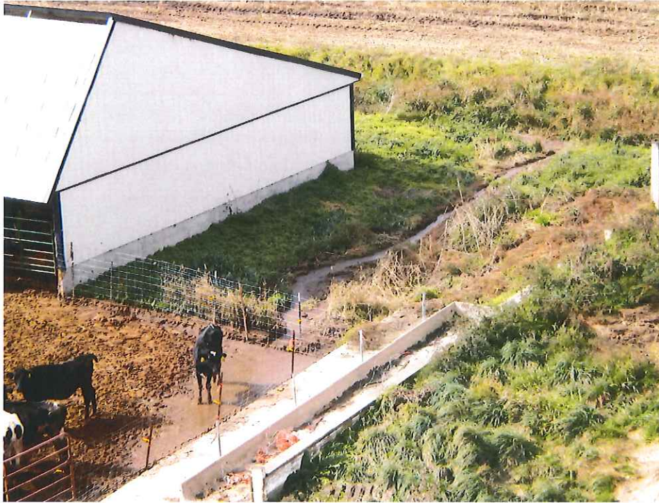
Concrete feedlot with direct runoff to surface waters
