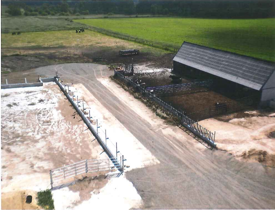
Viewing both concrete feedlots which are 100% contained with runoff being collected and pumped to long term storage. Zero discharge.
