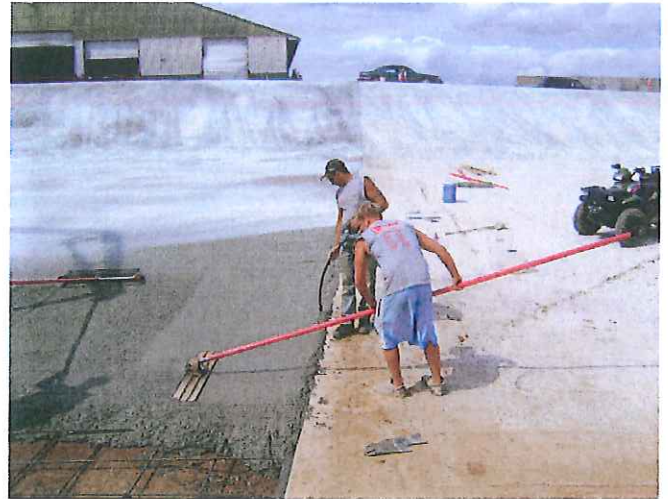
Waterstop joints bull floated and vibrated
