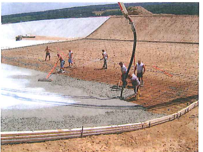
Subgrade was damped before concrete was installed
