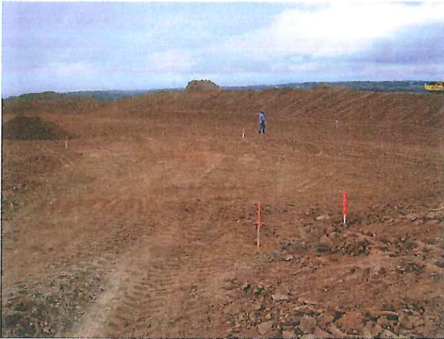
Final subgrade elevations
