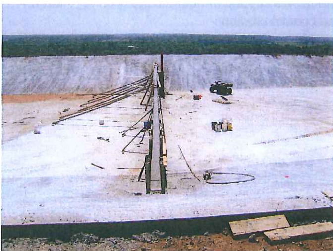
Separation wall formed with level control structure
