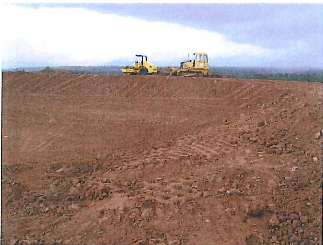
Completed subgrade and berms
