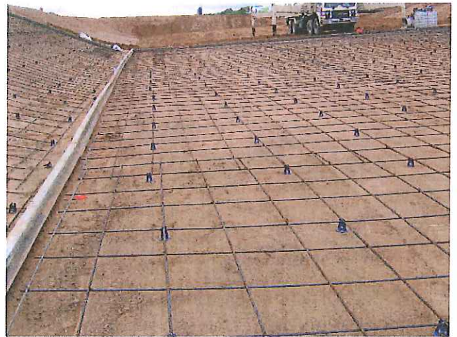
Plastic chairs set at every third rebar
