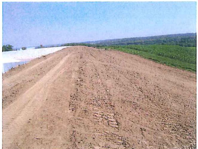
Top soil reapplied to berms and disturbed areas
