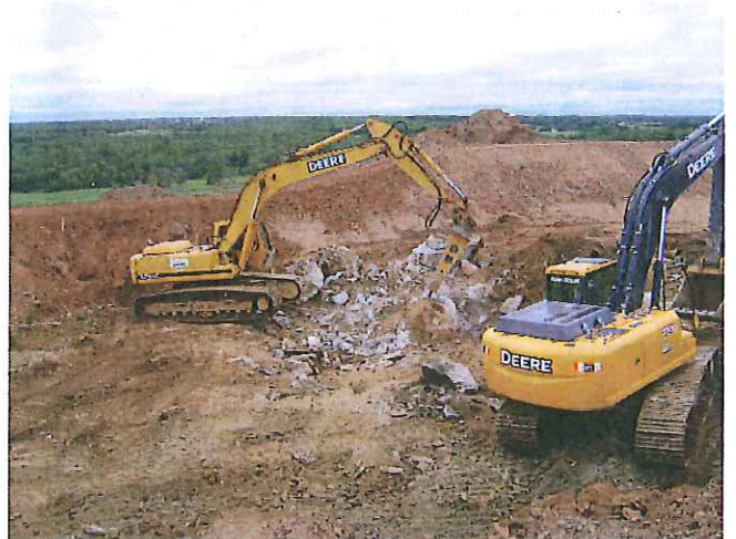
Bedrock being removed with hammer drill
