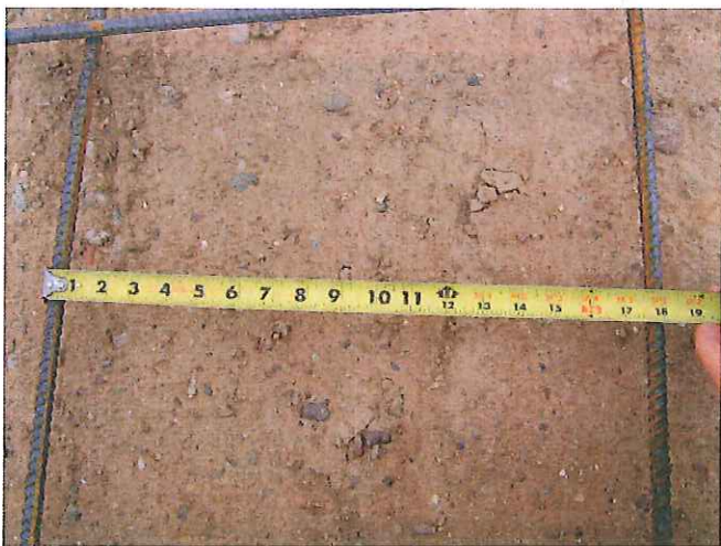
#4 grade 60 rebar spaced at 18" on center
