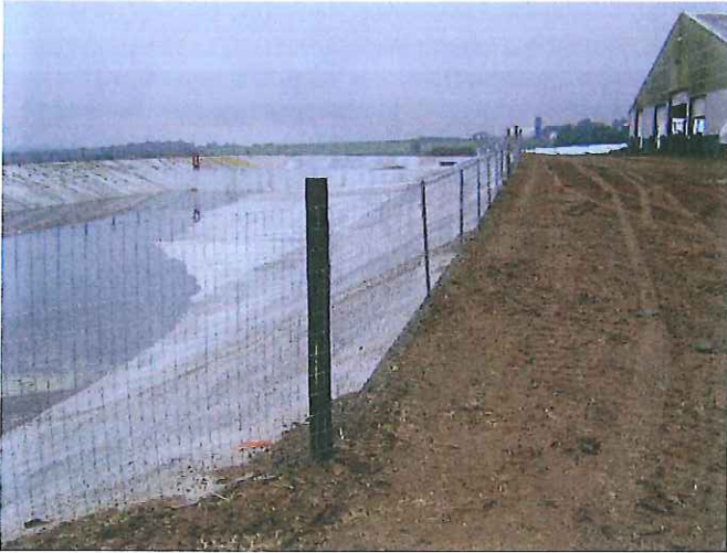
Fencing installed around manure storage facility
