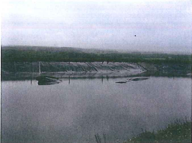
Original torn HDPE lined manure storage facility
