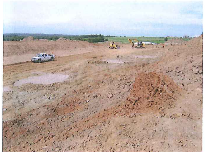
Water seepage areas were filled with \frac{3}{4} " stone
