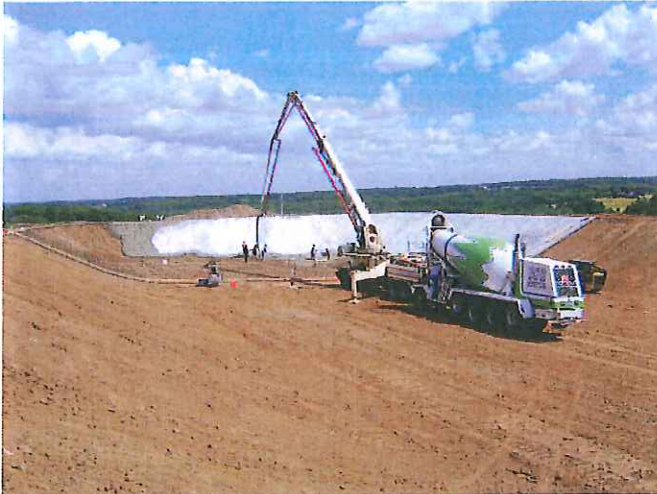
Concrete supplied by Morgan Sand & Gravel
