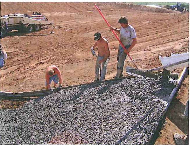
Installing concrete in waterstop form
