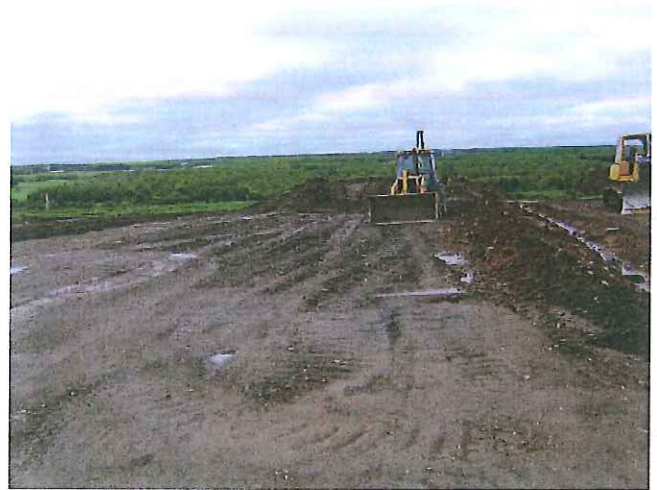
Top soil was removed for new manure storage facility foot print
