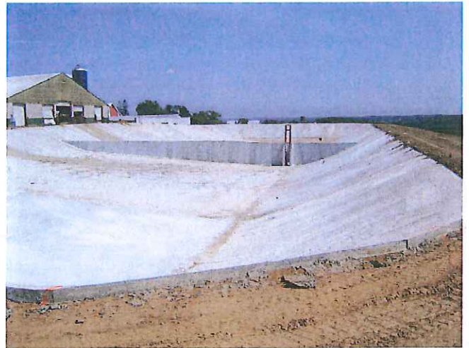
Concrete work completed
