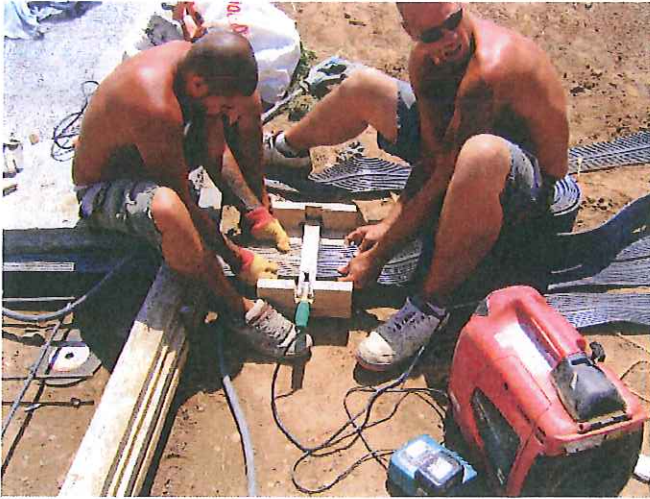
Waterstop butt weld
