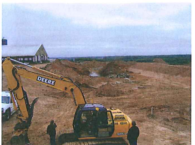
Bedrock was blasted and removed per NRCS state engineer
