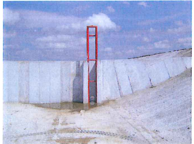
Level control structure installed in separation wall
