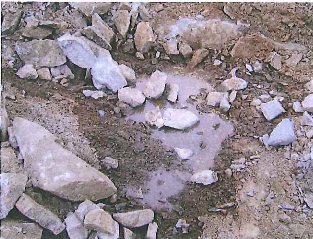
Water seepage after bedrock was blasted and removed
