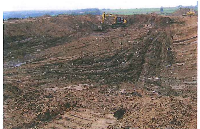
Contaminated soil removed and spread per nutrient management plan
