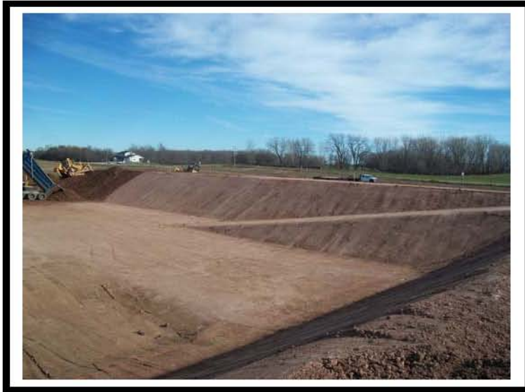
Photo #: 30 Photo Depicts: Pit construction Direction Pointed: Eastward
