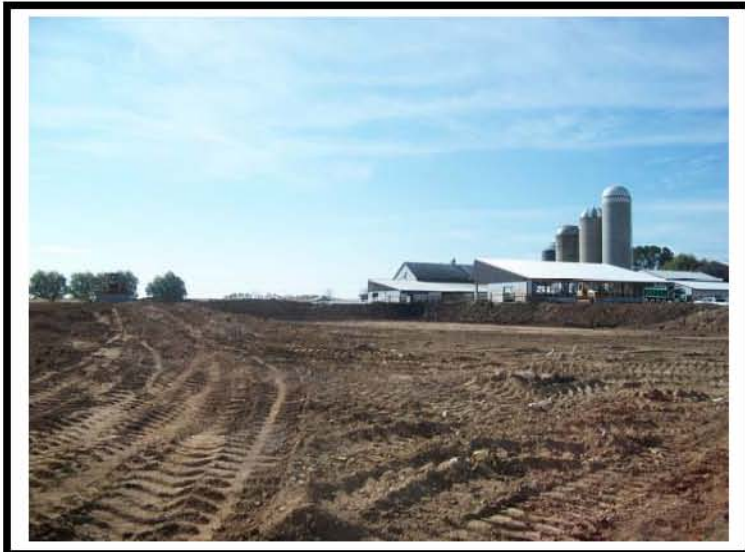
Photo #: 26 Photo Depicts: Pit construction
