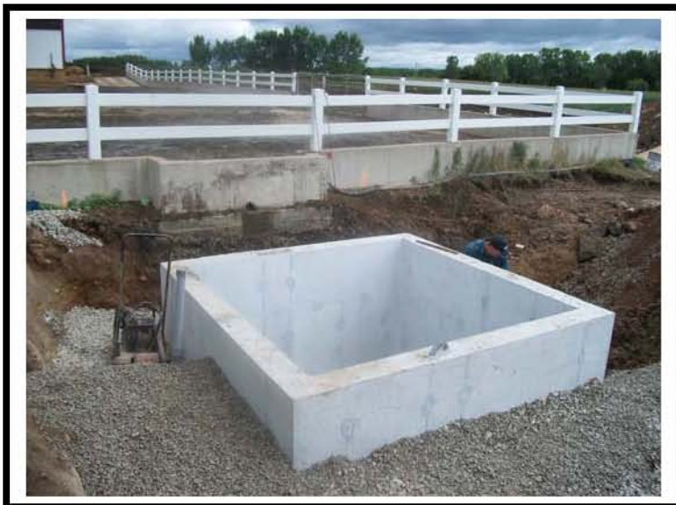
Photo #: 20 Photo Depicts: Tank construction
