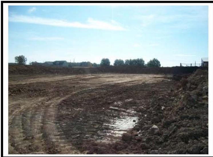
Photo #: 27 Photo Depicts: Pit construction
