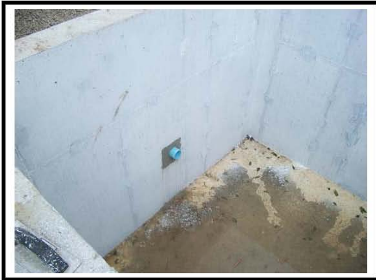
Photo #: 19 Photo Depicts: Tank Construction & transfer outlet from milkhouse tank.
