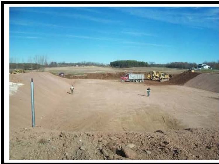
Photo #: 31 Photo Depicts: Pit construction Direction Pointed: Northward
