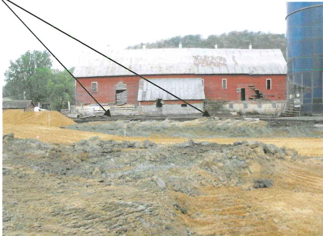
Barnyard Project under construction.
