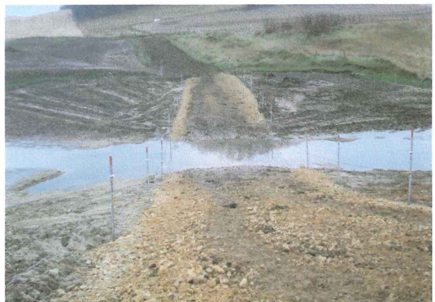
Completed crossing. Cattle are completely fenced out of the stream, except through the crossing.
