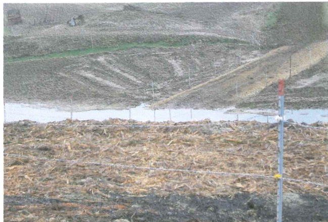
Completed crossing. Cattle are completely fenced out of the stream, except through the crossing.
