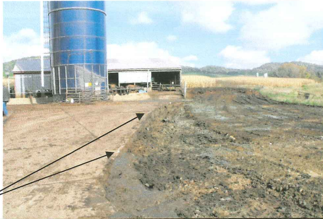
The concrete for the barnyard will tie into the existing concrete.
