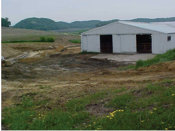
Barnyard site before construction
