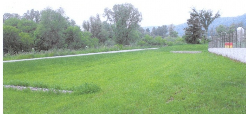
Area where the filter strip is located, from the spreader pad in the background to the washed rock located 1/2 way down filter strip shown in foreground. This was challenging because the family wanted the ability to be able to mow it with their lawn grass because of its proximity to the county road.
