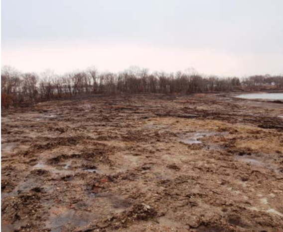
1 Sediment Placement Completed, 4/1/2011
