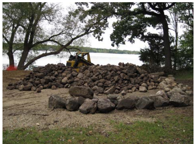
Left: Equipment access restricted to rock shelf to minimize disturbance to lakebed (9/2010) Right: Sand beach staging area for equipment access and stockpiling of materials
