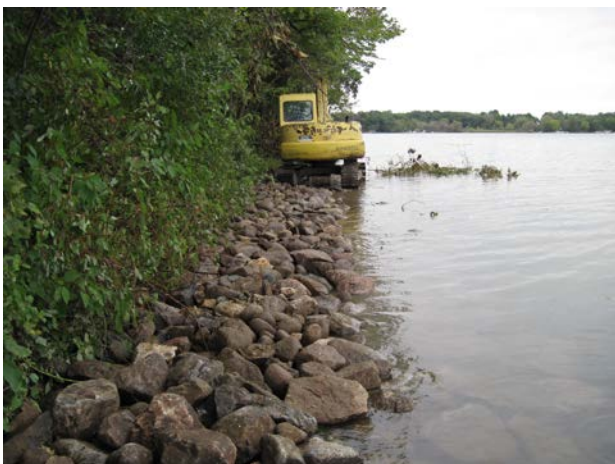
Left: Equipment access restricted to rock shelf to minimize disturbance to lakebed (9/2010) Right: Sand beach staging area for equipment access and stockpiling of materials
