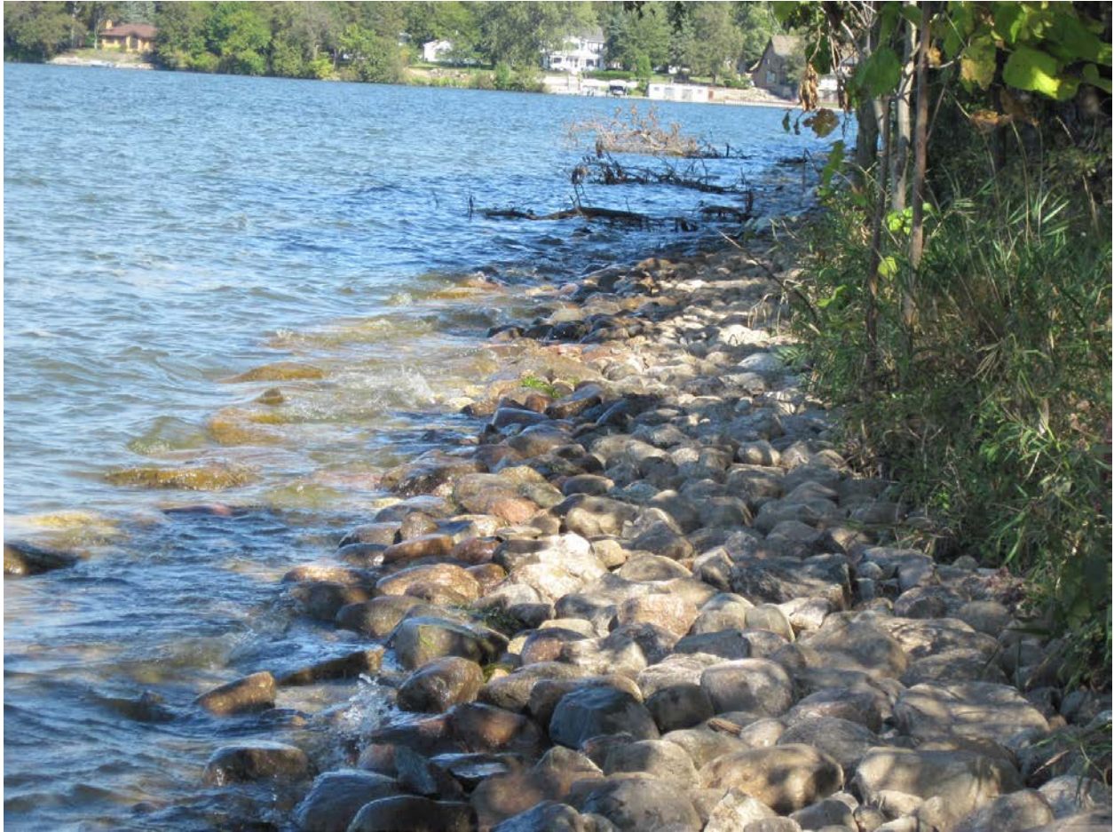
Picture of shoreline upon completion of riprap installation (9/2010)
