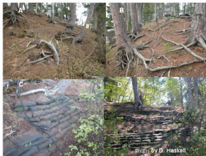
Figure 1. Photos A & B: before EnviroLok™ bags were installed. Photos C & D: after EnviroLok™ were installed on Moon Beach during the spring and summer of 2009.
