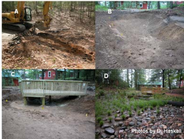
Figure 3. Construction of Rain Garden at Moon Beach in June of 2009. Photo A: asphalt being removed, photo B: excavation of rain garden, photo C: wooden bridge constructed over depression, Photo D: completed rain garden holding water during and after rain event.
