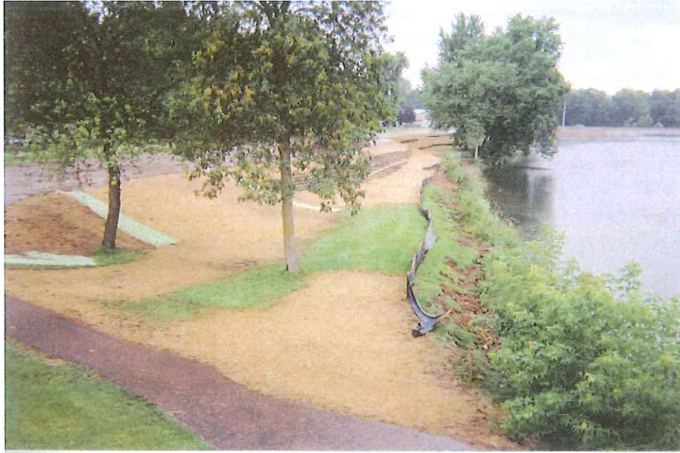
View of the south shore of Springville Pond, depicting the retaining wall and silt fence installed during the project.
