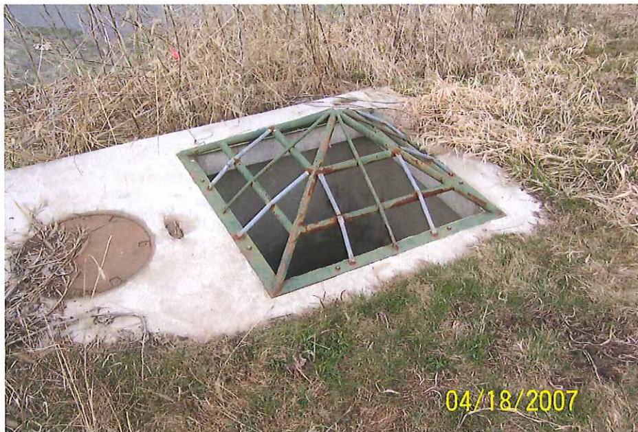
Post Project – Outlet Control Structure
