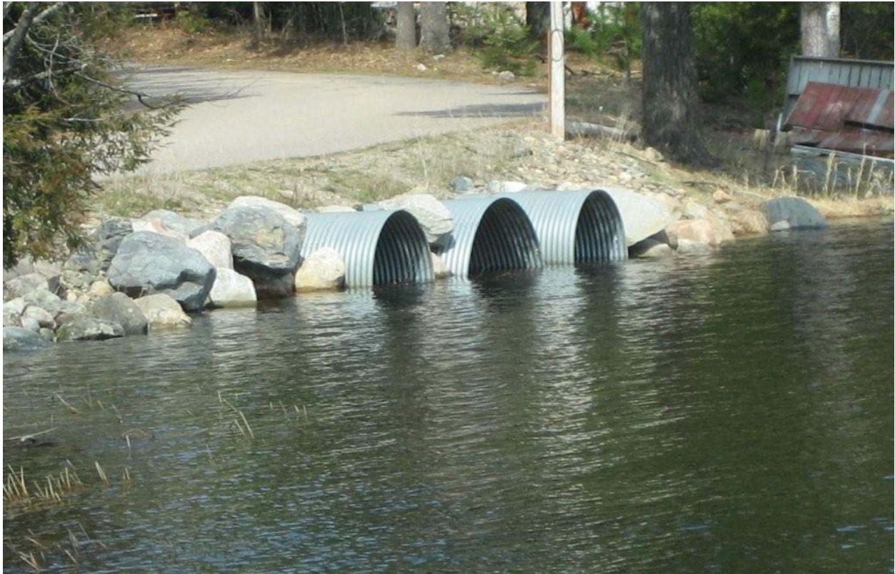
Photo 1. Culverts under Outlet Drive. The picture shows that the road may function as an earthen dam to control the boundaries of the lake, but flow is only minimally restricted by these three large culverts. This location is most likely the appropriate place to put a staff gauge.
