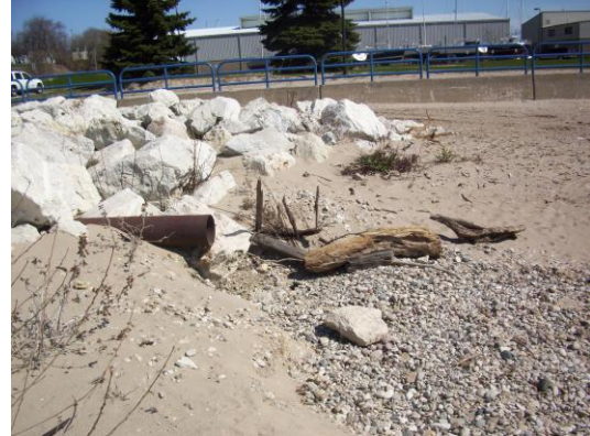
Photo 71: Stormwater pipe draining parking lot runoff onto YMCA Beach.
