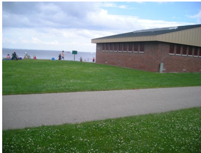
Photo 40: Looking east from behind Menominee Park Beach, showing turf grass and concession stand.
