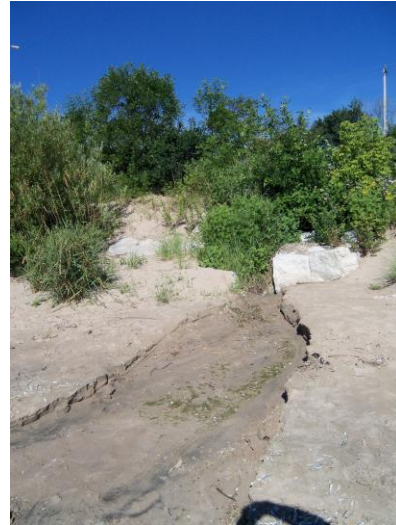
Photo 35: Stormwater outfall on the north end of Memorial South Beach.
