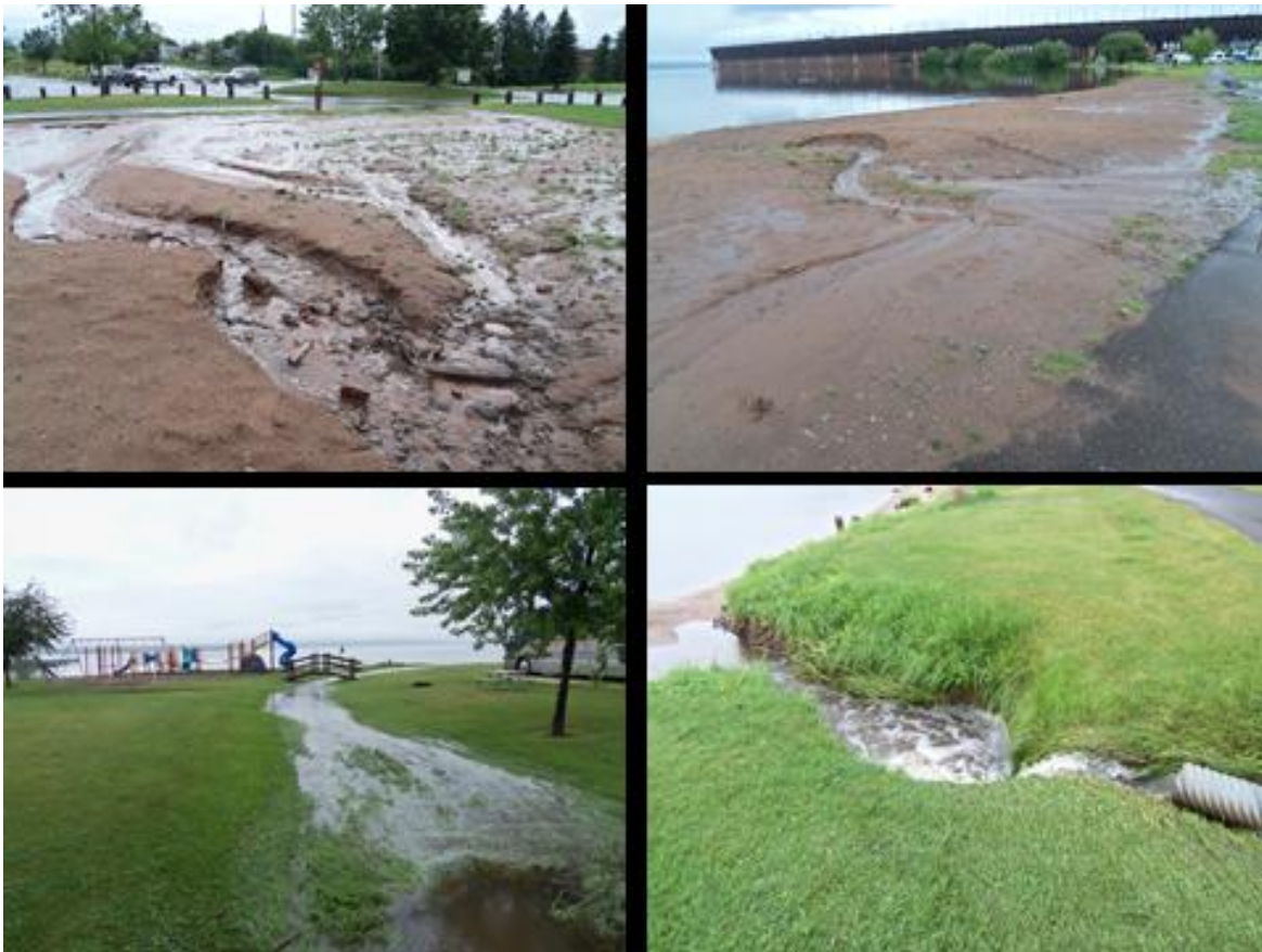
Photo 29: Kreher Park Beach after a significant rain event (>0.5 in) showing stormwater runoff.
