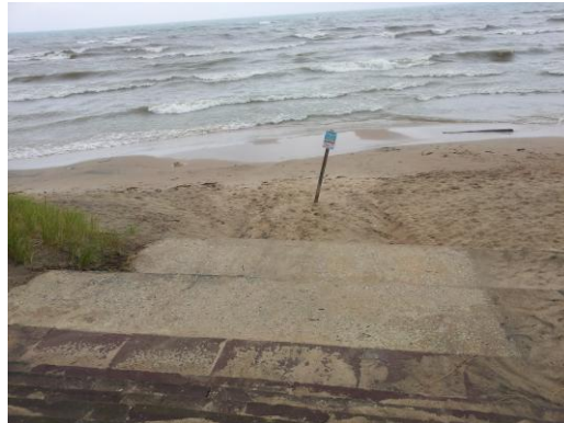
Photo 47: Looking from the concession building down onto the beach.
