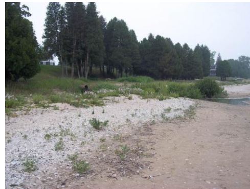
Photo 13: Looking north toward the southern stormwater outfall at Crescent Beach in the City of Algoma.
