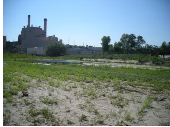
Photo 63: Stormwater discharge and coal power plant. Picture taken from beach proper looking onshore.
