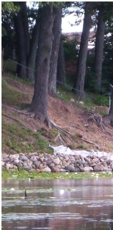
Figure 53. Erosion on shoreline.
