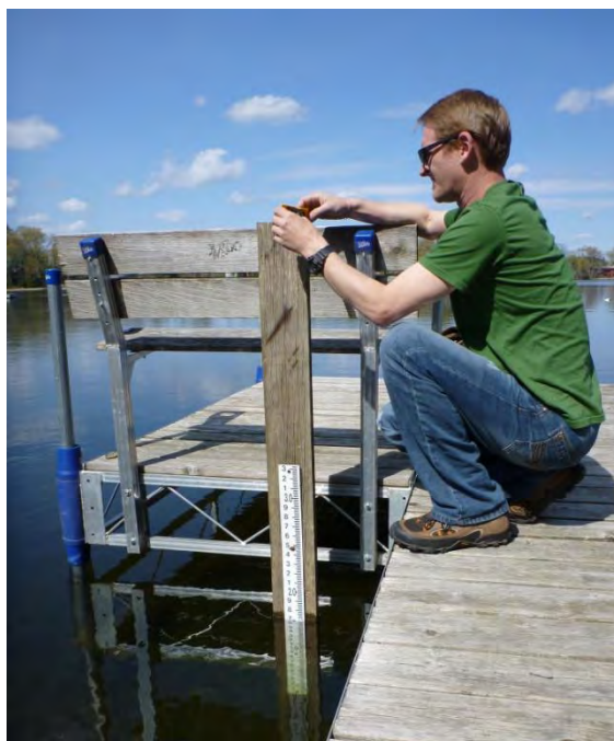
Figure 11. Installation of staff gauge.
