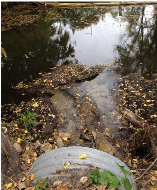
**FIGURE 3.2 SAND DEPOSITION AT THE CULVERT OUTLET INTO MILJALA CHANNEL. PHOTO CREDIT: STEVE NEARY, 10.5.12.**
